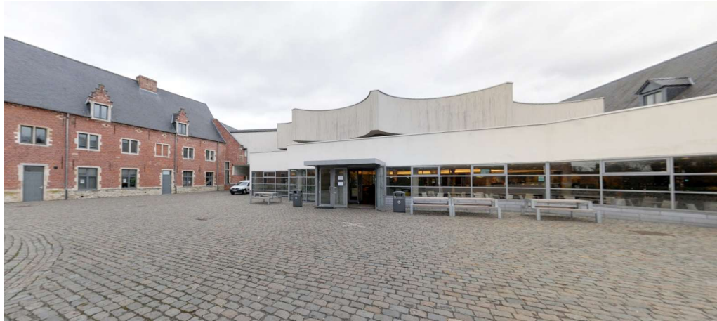
Figure 5.16 Arenberg Campus Library
