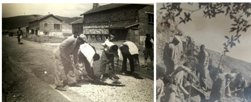
Figure 5.13. students were building and repairing roads
