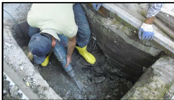
Figure 4.32. Maintenance of Sanitary Systems
