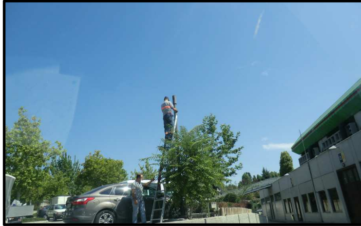
Figure 4.33. Electric Pole Maintenance
