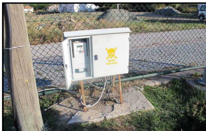
Figure 4.36. Distribution Board
