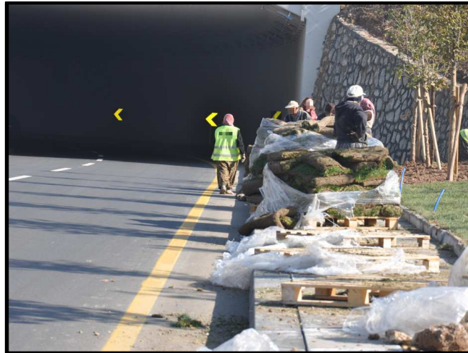
Figure 4.7. Preparation of Turf Laying on the Roadside
