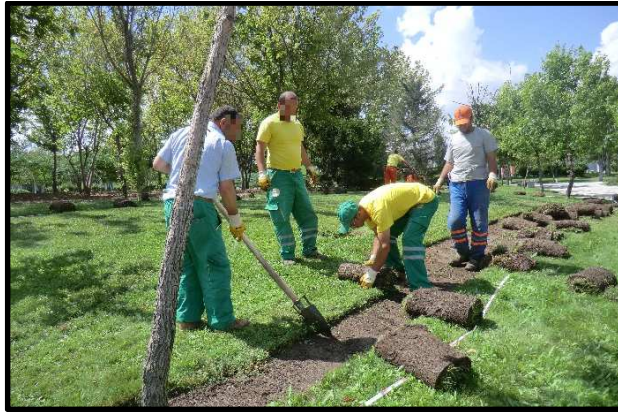
Figure 4.5. Turf Laying
