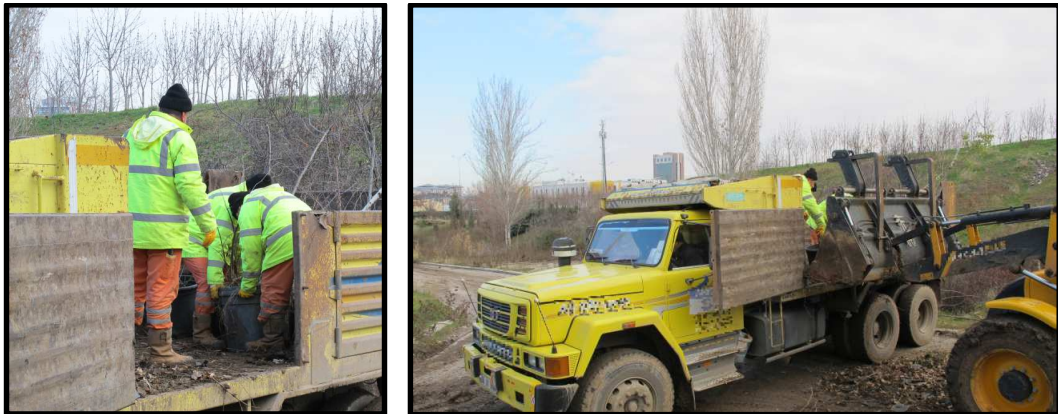
Figure 4.14. Lifting of Pots
