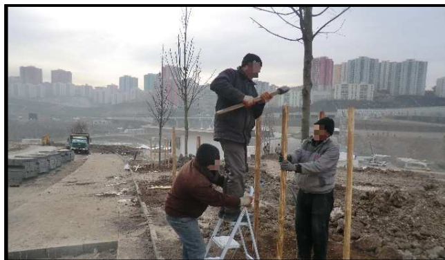
Figure 4.23. Penetrating Stakes into Soil
