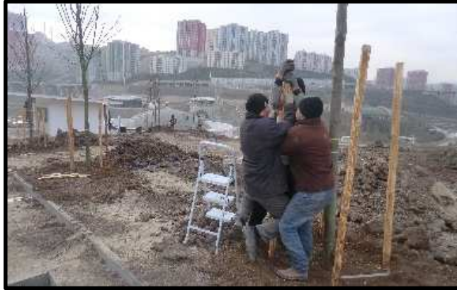
Figure 4.22. Placing Stakes into Ground
