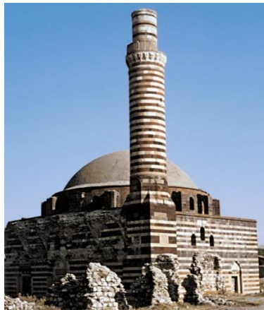
Figure 5.19. Hüseyin Paşa Mosque after partial restorations in 1975
