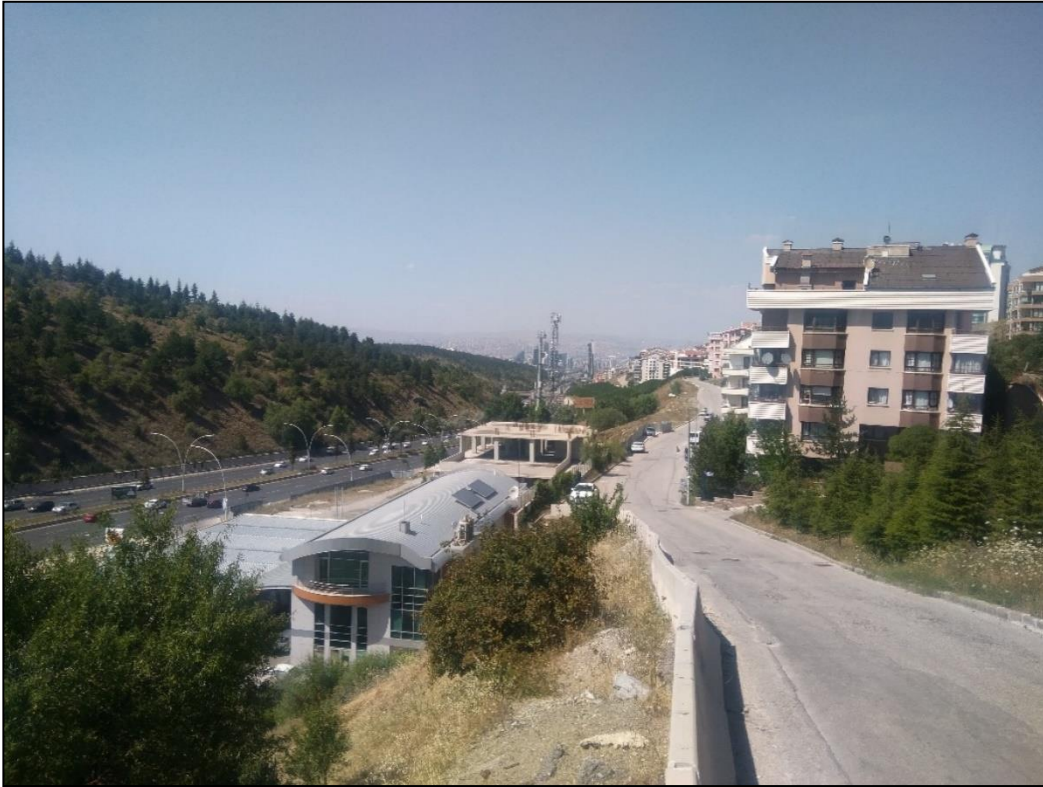
Figure 4.2. A view of the slope towards north (July 2019).
