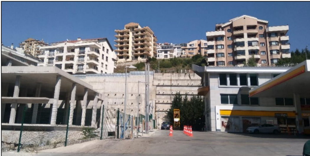
Figure 4.3. A view from the toe of the slope towards crest (July 2019).
