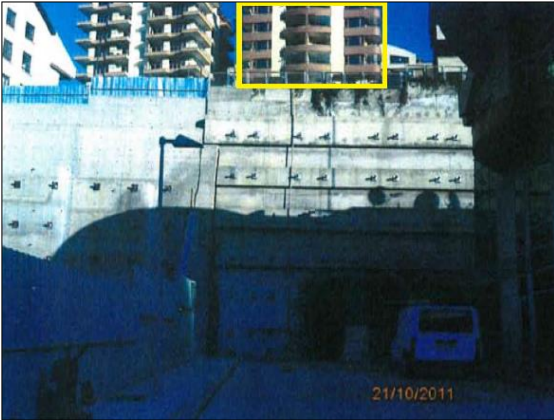
Figure 4.4 A view of Güneş Apartment from the downhill (Çokca et al., 2011).
