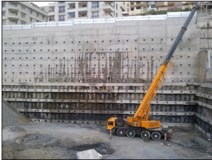
Figure 4.8. View of the business center foundation excavation and support system (Bakır, 2011).
