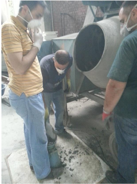
Figure 3.2 Slump Test is Performed with Rotary Mixer in the Background
