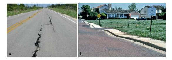
*Figure 2.1.* Expansive soil related problems. a- longitudinal cracks in road (Wang, 2016), b- heave in road and pavements (Colorado Geological Survey, n.d.)
