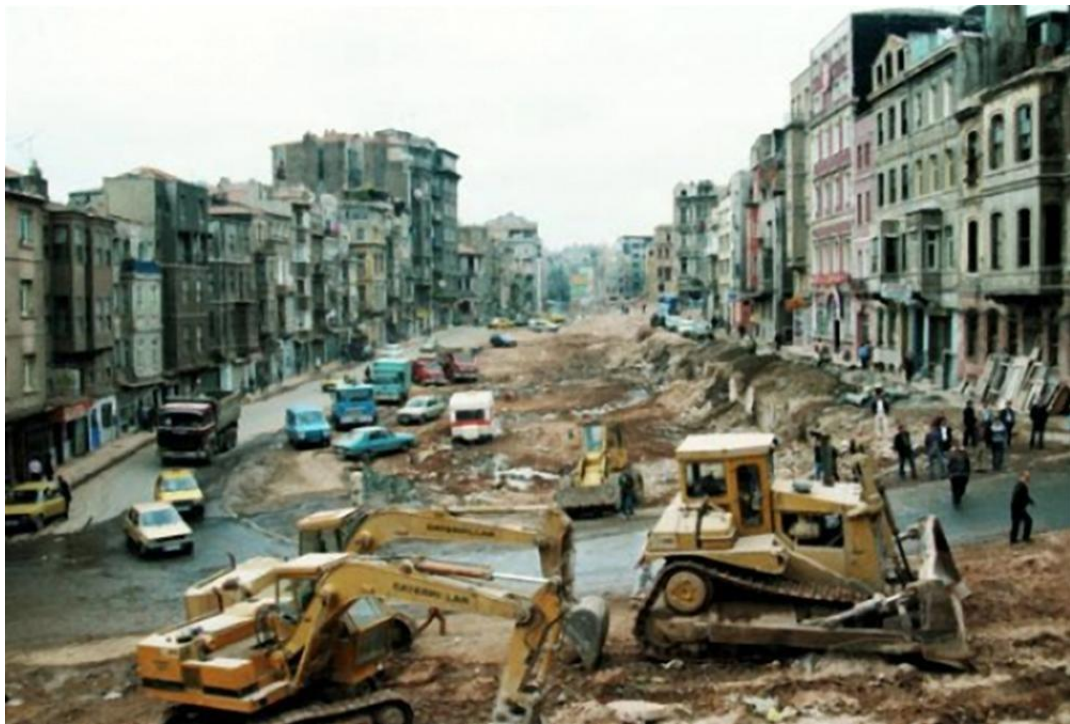
Figure 6. “Tarlabasi Demolitions” in the 1980s
