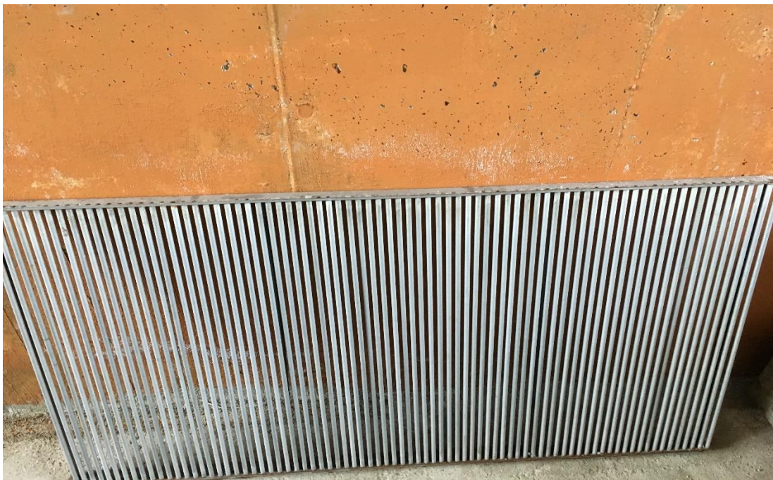
Figure 3.10. View of the rack with clear bar spacing of e_3=10 mm
