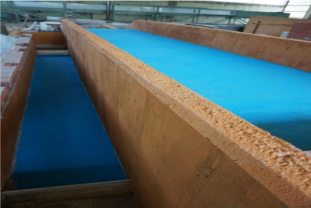
Figure 3.6. Downstream view of the “Intake Channel”
