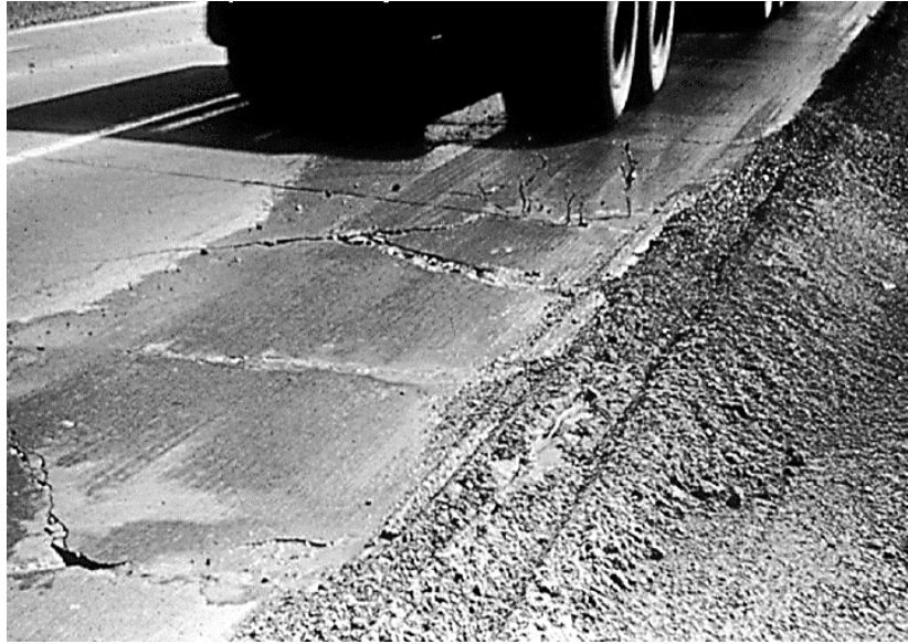
Figure 2.5. Pumping of fines (Arabzadeh. A., 2015)
