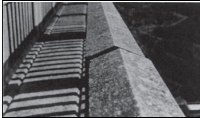
Figure 2.13 Parapet of Val de Mare Dam, Jersey [Poole, 1992]
