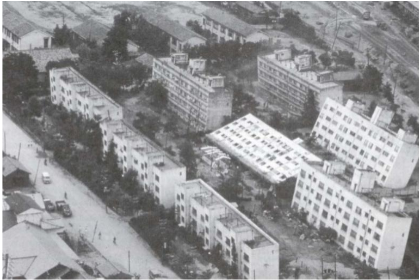
Figure 1.2. Foundation failure by liquefaction after the 1964 Niigata Earthquake (Kramer and Elgamal 2001)
