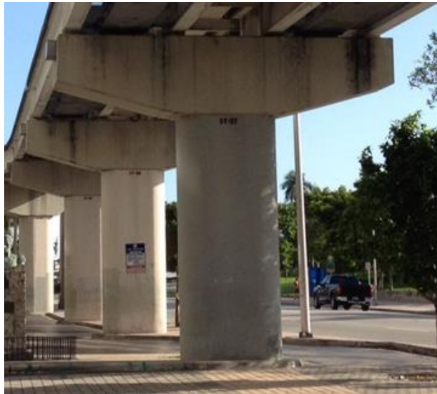
Figure 1.1. Hammer-head Pier Cap
