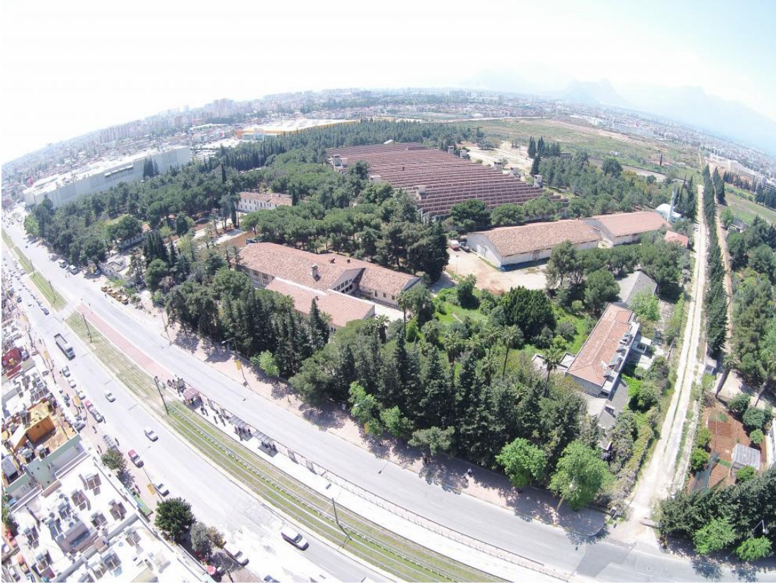
Figure 3.136. Cotton Weaving Factory, under restoration process, 2015. (Source: Kepez Municipality, http://www.kepez-bld.gov.tr/news.php?id=4184 )
