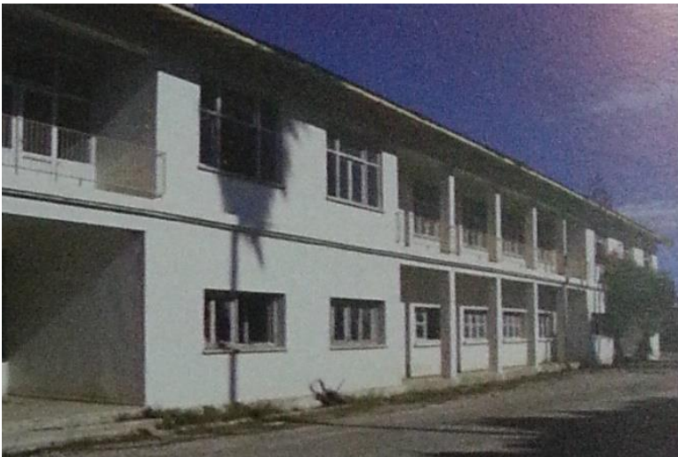
Figure 3.20. Administration building of the Hot Climate Botanic Experimental Station ( Sıcak İklim Nebatları Teksir ve Islah İstasyonu ) (Source: Çetin, 2012)
