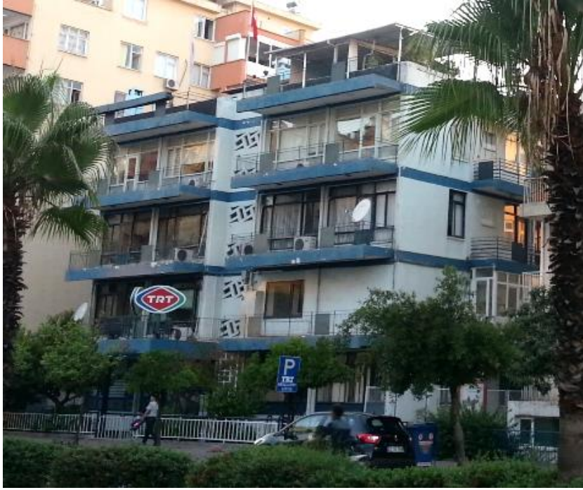
Figure 3.47. Turkish Radio and Television Association ( TRT ) building, built in 1970. (taken by the author, 2014)
