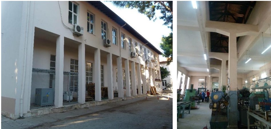
Figure 3.36. Antalya Boys' Art School, Block B and metal atelier, 1946. (taken by the author, 2013)
