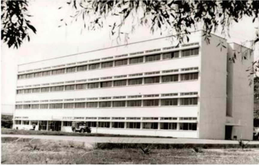
Figure 3.45. XIII. Regional Directorate of State Hydraulic Works (DSİ), 1967. (Source: Büyükyıldırım, 2017, p.363.)
