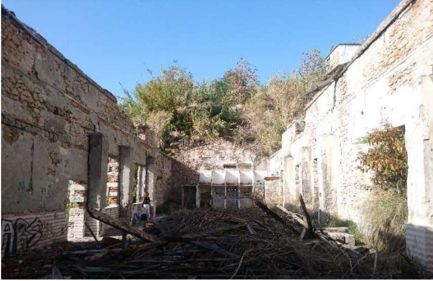
Figure 3.130. The interior space of Antalya Hydroelectric Plant. (taken by the author, 2017)
