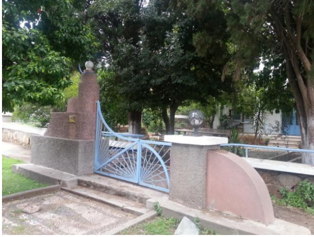
Figure 3.103. The main entrance of Villa Dr. Onat. (taken by the author, 2013)
