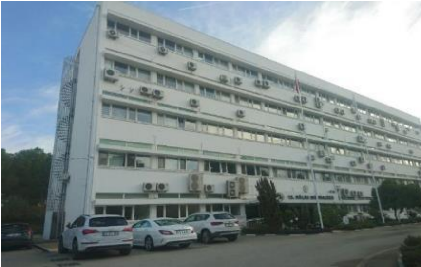
Figure 3.46. XIII. Regional Directorate of State Hydraulic Works (DSİ), built in 1967. (taken by the author, 2017)
