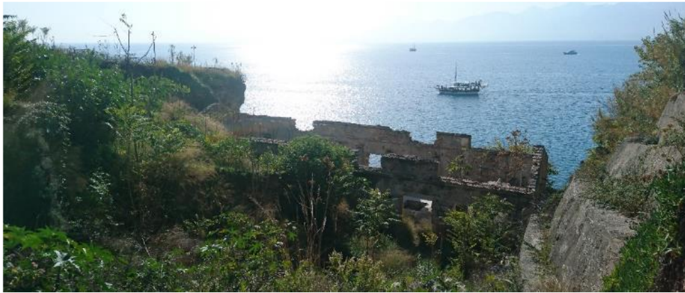
Figure 3.129. Top view of Antalya Hydroelectric Plant. (taken by the author, 2017)
