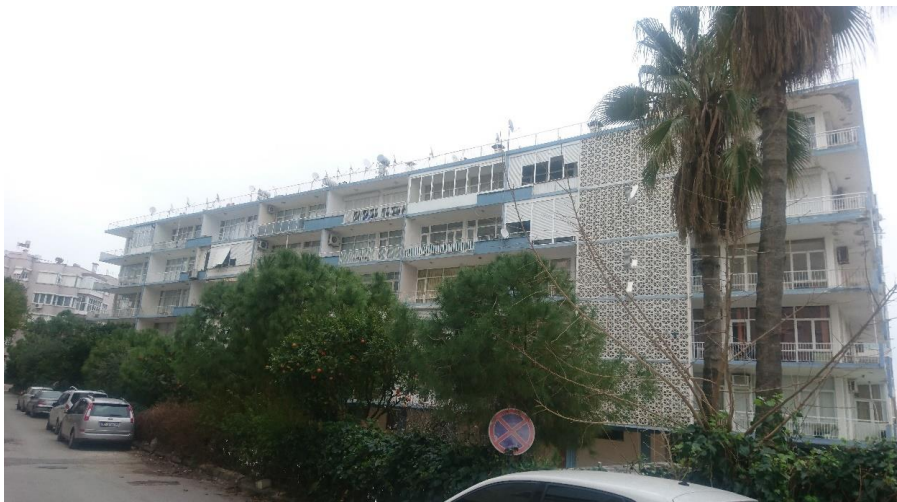
Figure 3.116. The general view of Yalı Apartment. (taken by the author, 2019)
