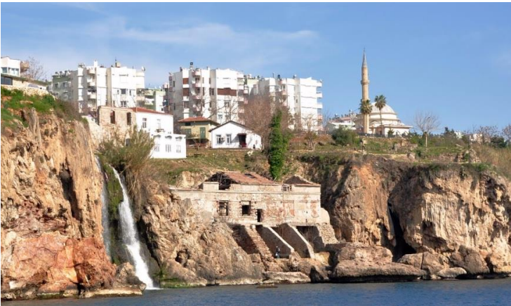
Figure 3.127. Antalya Hydroelectric Plant, established by Tevfik Işık. (Source: Google Maps, 2015)
