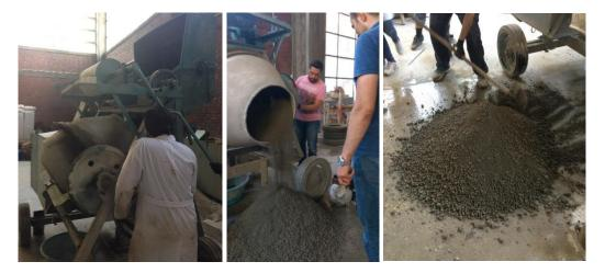
Figure 3.3. Mixing RCC mixture with rotary drum mixer and shovel on the ground
