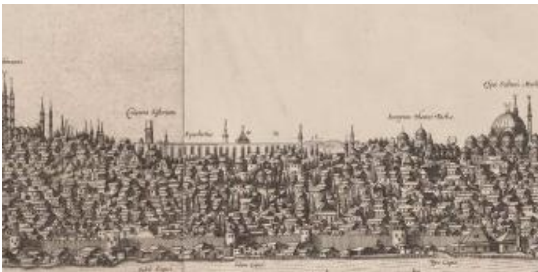
Figure 50.1: Detail showing the Valens Aqueduct.
