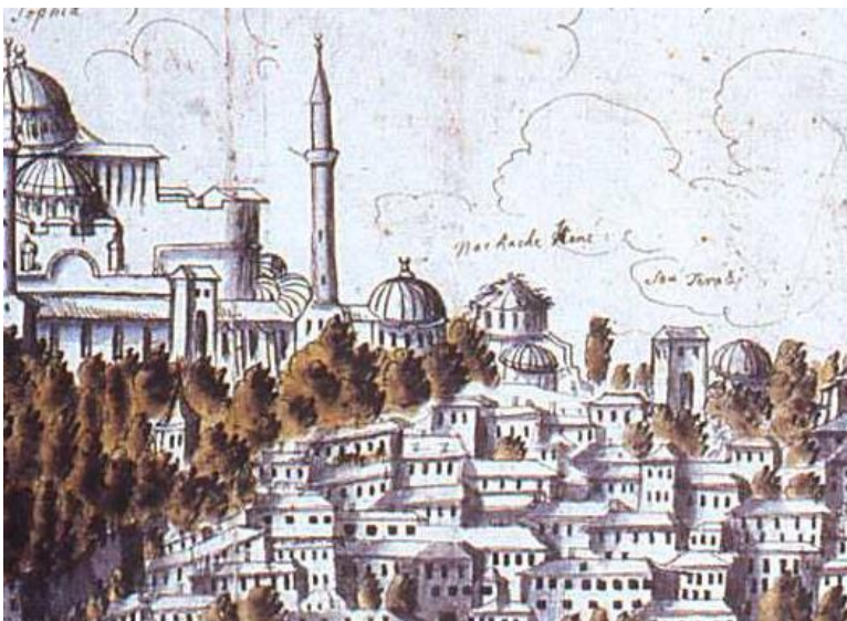
Figure 58: Detail from the panoramic view of Istanbul by Cornelius Loos, showing the water tower near Hagia Sophia with the inscription of “Sou Terasi”. Retrieved from https://twitter.com/recepkanal/status/962035604572618753?lang=fi
