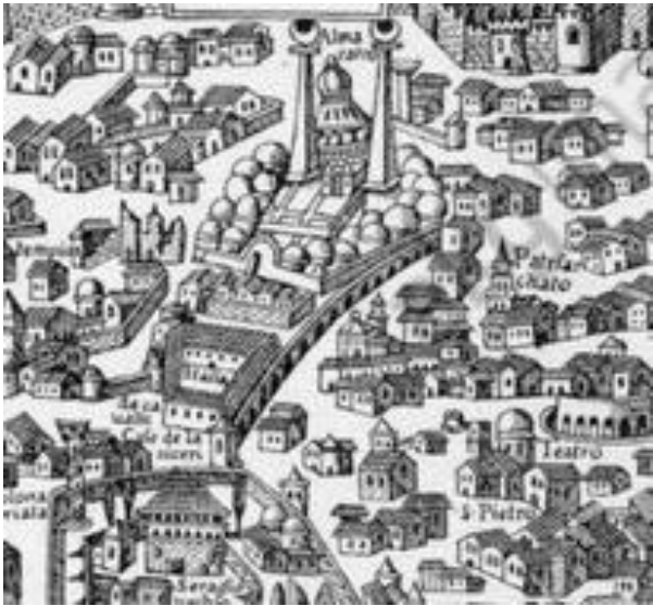
Figure 29.1: Detail showing the Aqueduct of Valens and its water tower.
