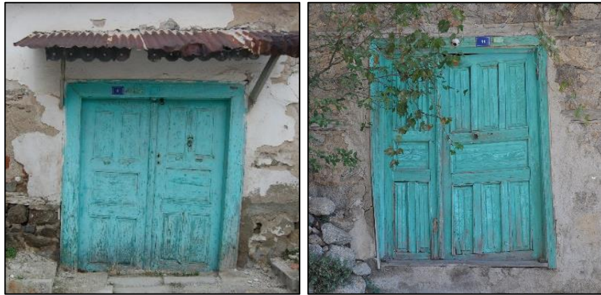
Figure 3.147. Exterior double wing panel doors located on stone masonry wall, exterior façades; Type 2 (Yenice N. b. block-lot: 11-16; right, Camikebir N. b. block-lot: 507-1)
