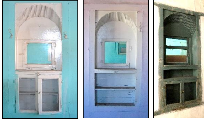
Figure 3.224. Examples of Cupboards on the timber framed wall (left, middle, Demirci N. b. block-lot: 443-13; right, Yenice N. b. block-lot: 521-7-8)
