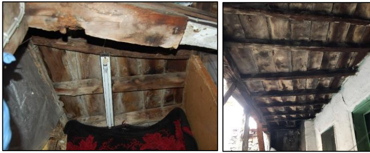
Figure 3.58. Simple timber flooring (Type 1) used in the sofa on the first floor (left, Demirci N. b.block-lot: 444-15; right, Kubbeli N. b.block-lot: 186-36)
