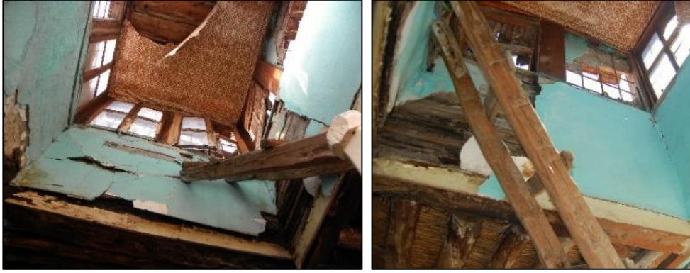
Figure 3.36. Timber framed wall covered with timber lath and then plastered (Kubbeli N. b.block-lot: 186-36)
