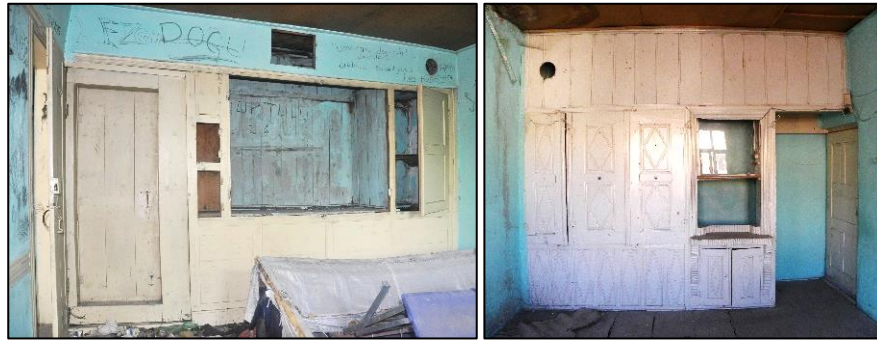
Figure 3.225. Examples of built in cupboards-yüklük (left, Cumhuriyet N. b. block-lot: 433-2; right, Demirci N. b. block-lot: 443-13)
