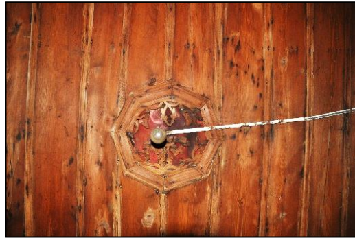
Figure 3.203. Timber ceiling covered with timber boards, timber laths and göbek at the center; Type 2B (Kılıç N. İsmet Çağlar Paşa St. N:34 b. block-lot: 170-44)
