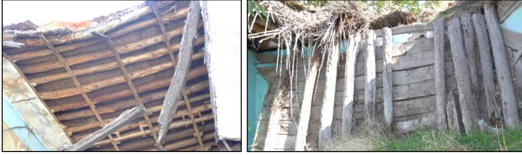
Figure 3.201. Timber ceiling covered with timber boards; use of timber girders in 2-3cm thickness (left) and use of timber boards (right) (left, Kubeli N. b. block-lot: 186-36; Cumhuriyet N. b. block-lot: 432-14)
