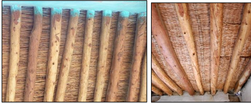
Figure 3.200. Timber ceilings that are not covered with timber boards in upper floor (Type 1B); without matting of straw (left), with matting of straw (right) (left, Demirci N. b. block-lot: 448-2; right, Camikebir N. b. block-lot: 196-1)
