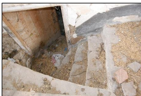
Figure 3.134. Stone stair provide access to the basement floor from taşlık; Type1 (Yenice N. b. block-lot: 521-12)
