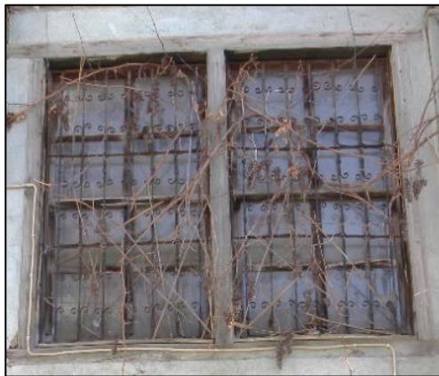
Figure 3.187. Example of double sash windows located on sofa (Demirci N. b. block-lot: 443-13)
