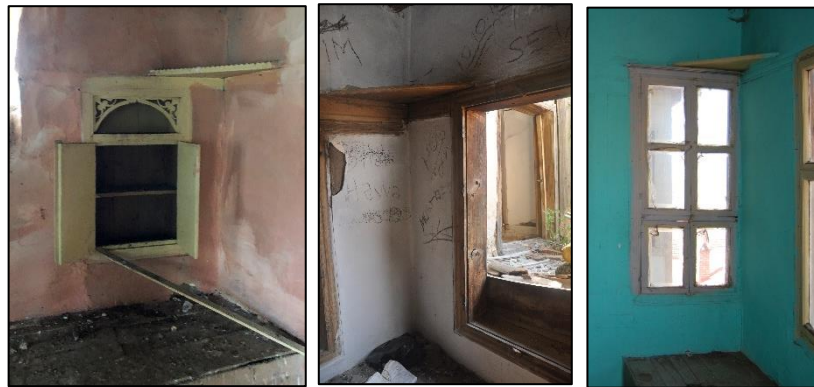
Figure 3.231. Examples of timber triangle shelves located corner above the cupboard (left), above the window (middle and right) (left, Kubbeli N. b. block-lot: 186-36; middle, Cumhuriyet N. b. block-lot: 433-2; right, Demirci N. b. block-lot: 443-13)
