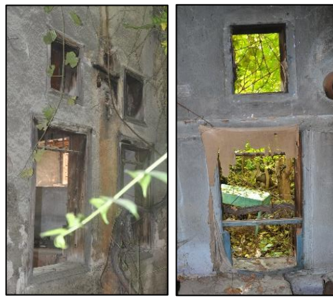
Figure 3.183. Window opening with top window on timber framed wall; Type 6 (Cumhuriyet N. b. block-lot: 433-3)
