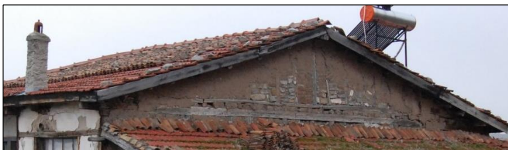
Figure 3.81. Example of gable wall (Yenice N. b.block: 521-7-8)
