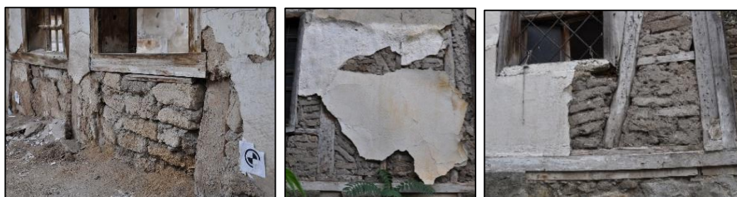
Figure 3.31. Timber framed wall with mudbrick infill (Kılıç N. b.block-lot: 170-44)
