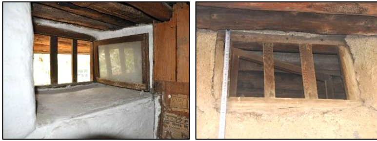
Figure 3.176. Top window opening located in the middle and above the two niches on stone masonry wall; Type 4 (Cumhuriyet N. b. block-lot: 433-2)
