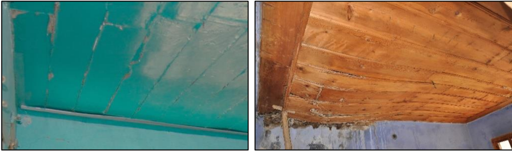
Figure 3.202. Timber ceiling covered with timber boards; Type 2A (left), timber ceiling covered with timber boards and timber laths, Type 2A (right) (left, Yenice N. b. block-lot: 11-16; right, Kılıç N. b. block-lot: 170-19)
