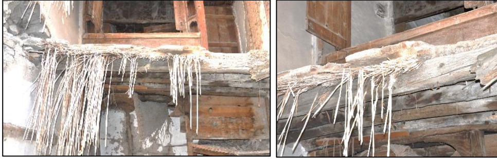
Figure 3.72. View of layers of flooring, Type 2, with terracotta tiles used in room (Kılıç N. b. block-lot: 170-44)
