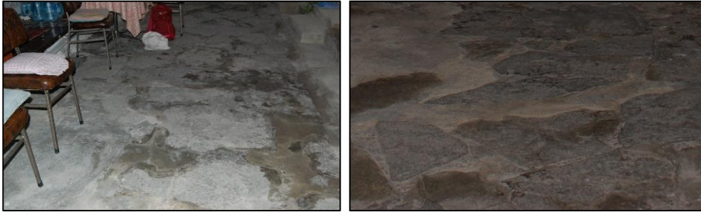
Figure 3.193. Stone pavement intervened with floor screed in taşlık space (Yenice N. b. block-lot: 521-12)
