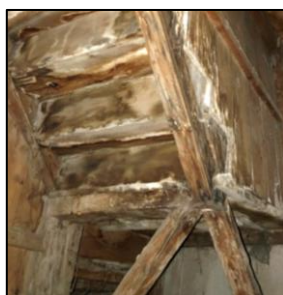
Figure 3.139. Lower connection of stringers supported by timber posts (Kubbeli N. b.block-lot:186-36)
