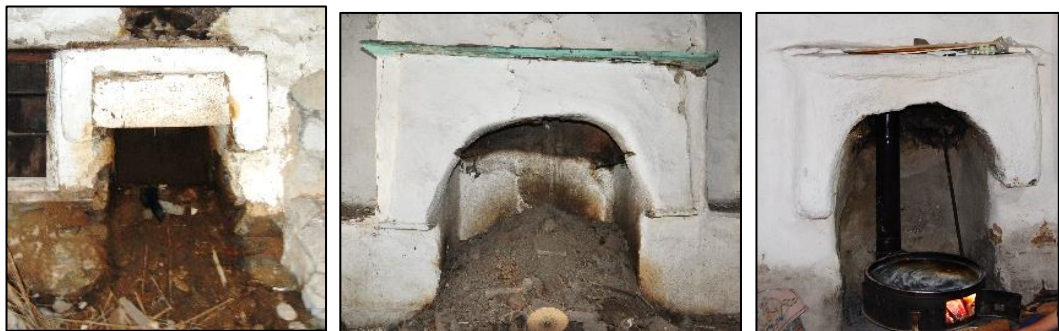
Figure 3.210. Fireplaces that have projected front face with arched shaped openings, Type 2B (left, Yenice N. b. block-lot: 12-30; middle, Cumhuriyet N. b. block-lot: 433-2; right, Demirci N. b. block-lot: 444-15)
