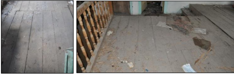
Figure 3.194. View of timber floor covering constructed with simple timber flooring used in the sofa (Cumhuriyet N. b.block-lot:433-2)
