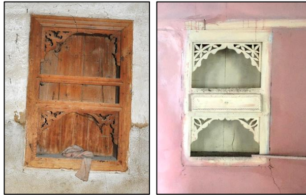
Figure 3.215. Niche located on the stone masonry wall and covered with timber boards, Type 1B (left, Kılıç N. b. block-lot: 170-4;right, Kubbeli N. b. block-lot: 186-36)
