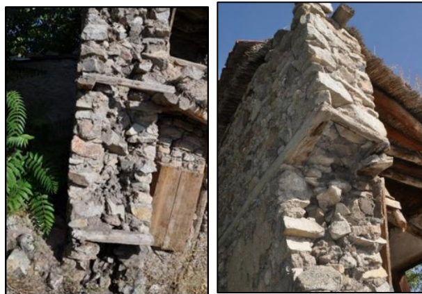
Figure 3.19. Stone masonry wall with timber lintels and tie beams (Gedik N. b.block-lot: 362-19)
