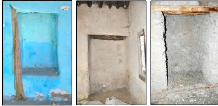
Figure 3.214. Niche located on the stone masonry wall, Type 1A (left, Kubbeli N. b. block-lot: 186-36; middle, Cumhuriyet N. b. block-lot: 433-2; right, Camikebir N. b. block-lot: 188-4)
