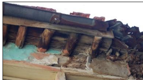
Figure 3.86. Timber eave covered with eaves fascia board-Type 2A (Kubbeli N. b.block-lot:186-36)
