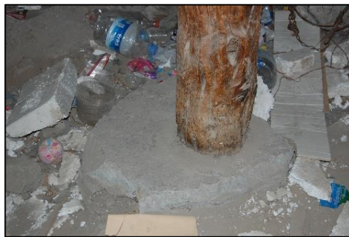
Figure 3.46. Stone base of timber post (Demirci N. b.block-lot: 448-2)
