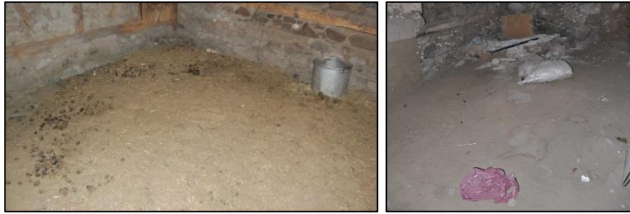
Figure 3.192. Pressed earth floor of entrance (left), of izbe (right) in ground floor (left, Cumhuriyet N. b. block-lot: 433-3; right, Cumhuriyet N. b. block-lot: 433-2)
