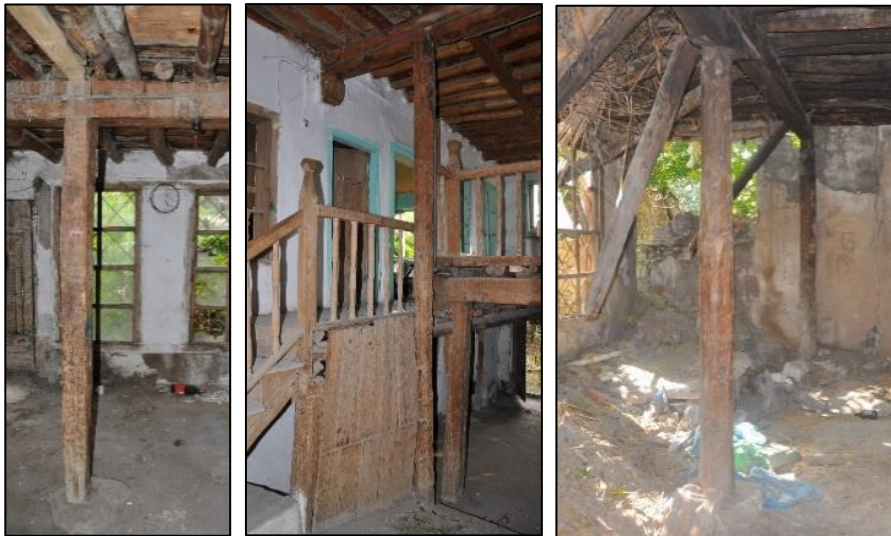
Figure 3.39. Timber posts used in ground floor (Cumhuriyet N. b.block-lot: 433-2)
