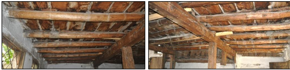
Figure 3.62. Simple timber flooring (Type 1) used in the sofa on the mezzanine floor (Cumhuriyet N. b.block-lot:433-2)
