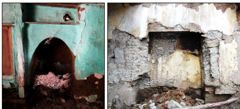
Figure 3.207. Fireplace with plain front face; Type 1A (left); Type 1B (right) (left, Kubbeli N. b. block-lot: 186-36; right, Yenice N. b. block-lot: 521-12)
