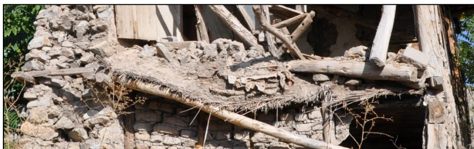
Figure 3.63. Flooring (Type 2) used in the room in first floor (Gedik N. b.block-lot:362-19)
