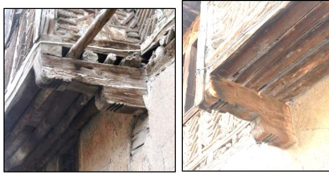
Figure 3.128. Examples of projections with overlapped beams, Type 2 (Cumhuriyet N. b. block-lot: 433-2)
