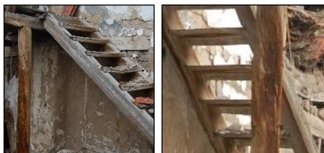
Figure 3.138. Timber step boards are placed into opened grooves on stringers-Type2B (Yenice N. b.block-lot: 12-30)
