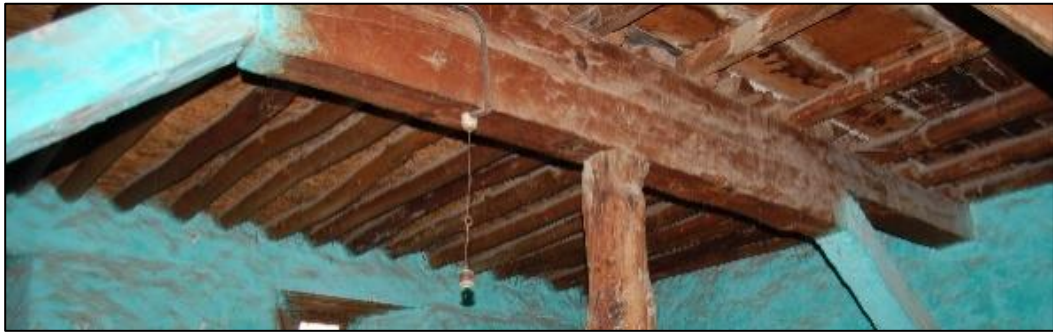
Figure 3.45. Type 2 - timber post with bolster on top (Demirci N. b.block-lot: 448-2)
