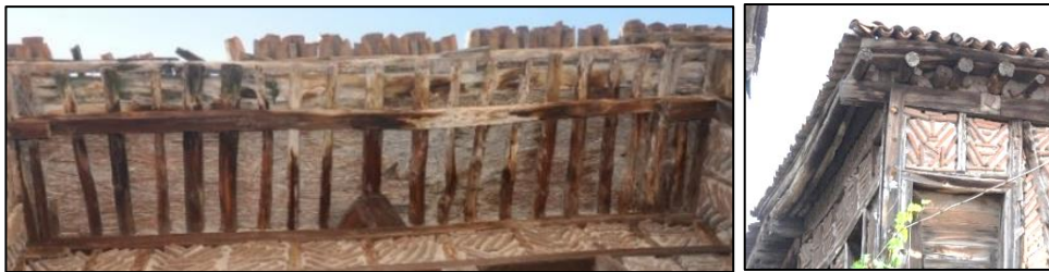
Figure 3.84. View of eave that is not covered-Type 1 (Cumhuriyet N. 2 b.block-lot: 433-2)
