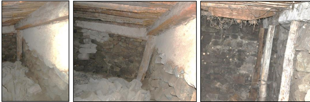
Figure 3.57. Timber floor beams supported by girder located on timber posts adjacent to the basement floor wall (left, middle, Kubbeli N. b.block-lot:186-9; right, Kubbeli N. b.block-lot:186-40)
