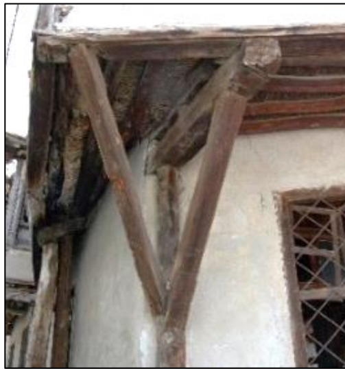
Figure 3.41. Type 1 – timber post with timber braces under the projection on the street façade (Camikebir N. b.block:196-1)
