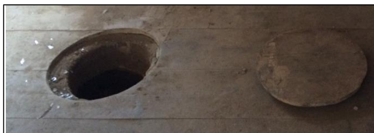
Figure 3.206. Tandır located on the floor of the room (Yenice N. b. block-lot: 11-16)
