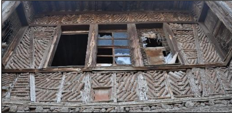
Figure 3.33. Timber framed wall with brick infill without plaster (Cumhuriyet N. b.block-lot:433-2)
