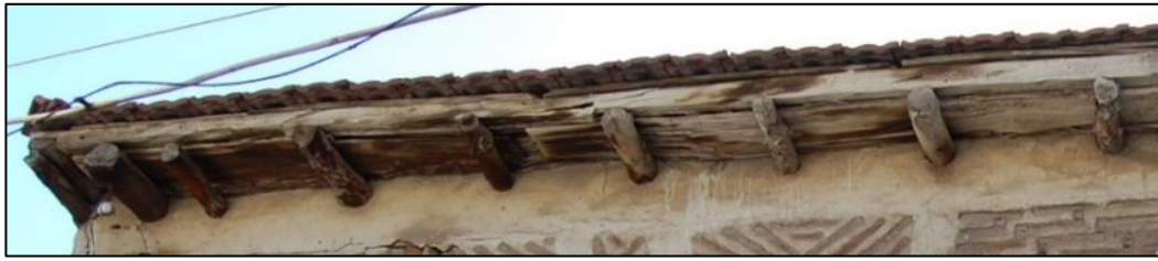
Figure 3.83. View of eave that is not covered-Type 1 (Demirci N. b.block-lot: 448-2)
