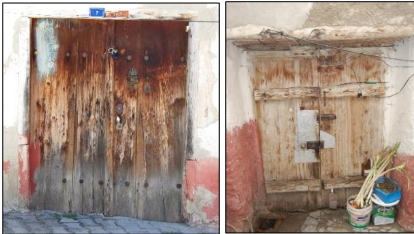
Figure 3.146. Exterior double wing batten door located on stone masonry wall; exterior facade (left), interior facade (right); Type 2 (Demirci N. b. block-lot: 444-15)
