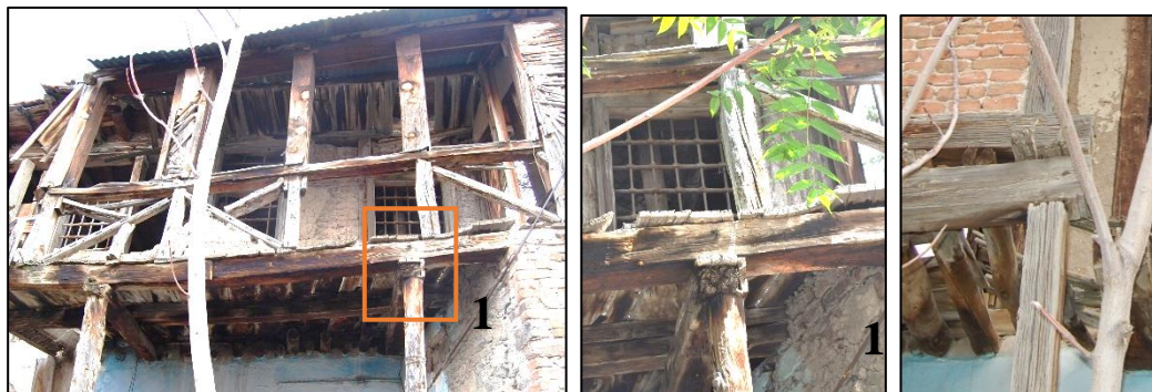
Figure 3.117. Connection detail 5, view of timber posts used in both floor (Kubbeli N. b.block-lot: 186-9)
