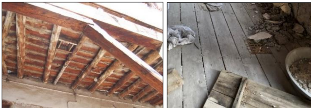
Figure 3.196. View of simple timber flooring (Type 1) with peep hole (Camikebir N. b.block-lot: 196-1)
