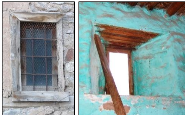
Figure 3.171. Window opening located on masonry wall; Type 2 (Demirci N. b. block-lot: 448-2)
