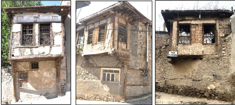
Figure 3.121. Projection types according to their forms, respectively; rectangular, trapezoid, triangle (left b. block-lot: 229-6; middle b. block-lot: 186-9; right b. block-lot: 228-17)
