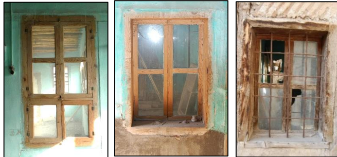
Figure 3.180. Window opening Type 5, Casement Windows (Demirci N. b. block-lot: 448-2)
