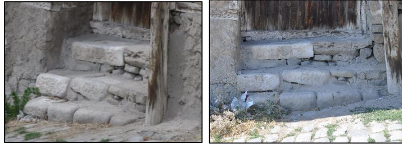
Figure 3.132. Stone stair used at the street entrance; Type1 (Kılıç N. b. block-lot: 170-19)
