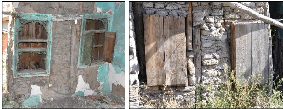
Figure 3.223. Cupboards on the timber framed wall, front face (left), rear face (right) (Gedik N. b. block-lot: 362-19)
