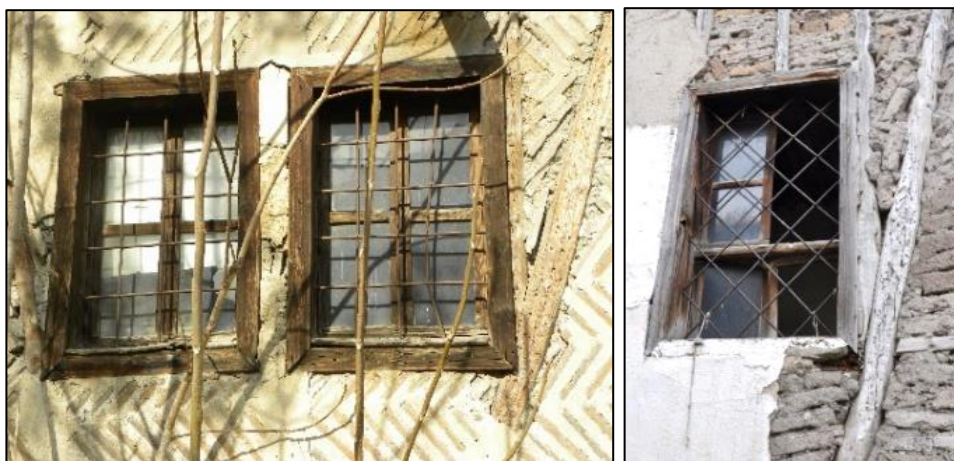
Figure 3.185. Examples of casement windows (left, Demirci N. b.block-lot: 448-2; right, Kılıç N. b.block-lot: 170-44)
