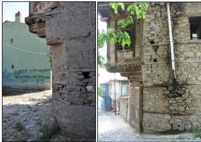
Figure 3.24. Examples of corner chamfer (left, Cumhuriyet N. b.block-lot: 433-3; right, Camikebir N. b.block-lot: 186-9)
