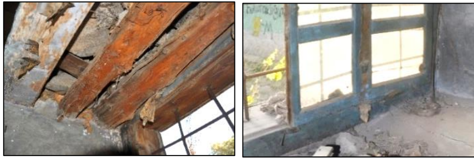
Figure 3.173. Detail of window opening located on stone masonry wall; Type 3 (Cumhuriyet N. b. block-lot: 433-3)
