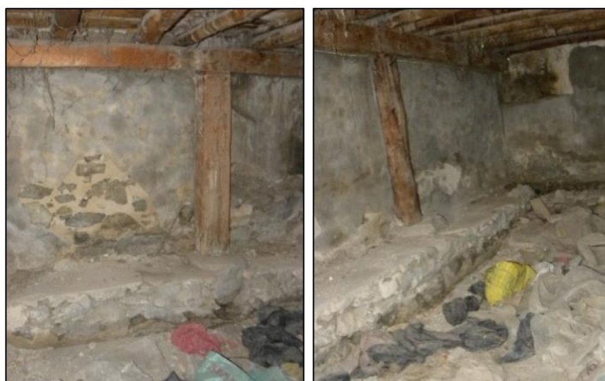
Figure 3.8. Continuous foundation with gradually decreasing width at one level at one side (Yenice N. b.blok-lot: 521-12)
