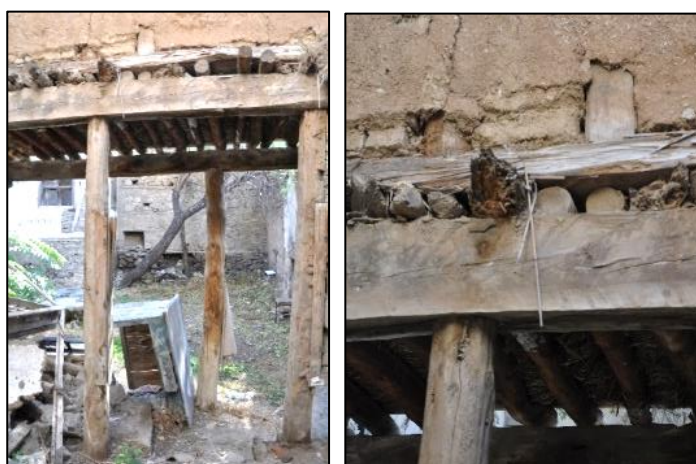
Figure 3.114. Connection detail 4, view of timber floor beams located on the wall plates of timber post (Kılıç N. b. block-lot: 170-44)
