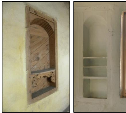
Figure 3.219. Niche with arch located on the timber framed wall Type 2B; (left, Demirci N. b. block-lot: 448-2; right, Kılıç N. b. block-lot: 170-19)
