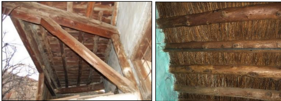
Figure 3.195. Bottom view of simple timber flooring -Type 1 (left), bottom view of flooring consist of layers – Type 2 (right) (Camikebir N. b. block-lot: 196-1)
