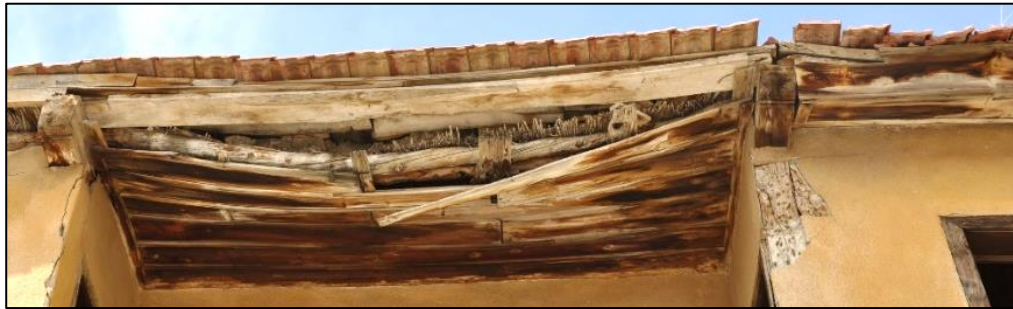
Figure 3.88 Timber eave covered with eaves fascia board and soffit board-Type 2B (Kılıç N. St. b.block-lot: 170-19)
