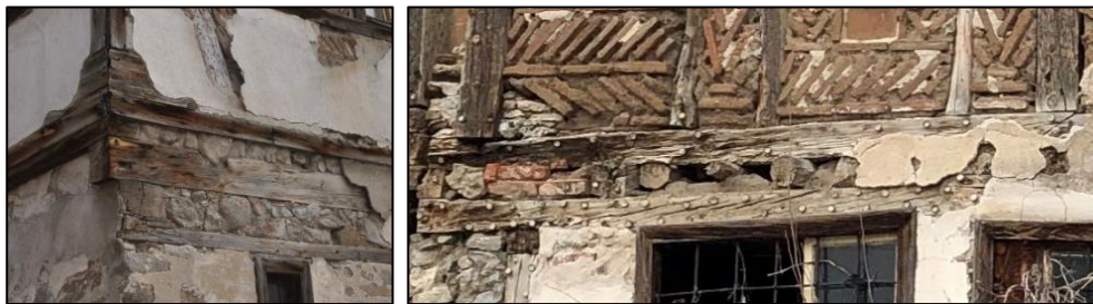
Figure 3.99. Connection detail 2, view of timber floor beams located on the wall plate of masonry wall in lower floor and foot plate located on the floor beams, timber posts set on the foot plate (left, Elmalı N. b. block-lot: 230-5; right, Yenice N. b. block-lot: 8-8)
