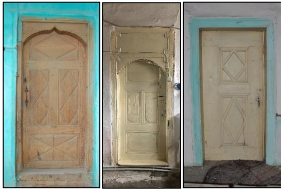
Figure 3.156. Example of interior single wing panel doors located on timber framed wall, Type 4; exterior view; (left, Demirci N. b. block-lot: 448-2; middle, Yenice N. b. block-lot: 521-7-8; right, Cumhuriyet N. b. block-lot: 433-2)
