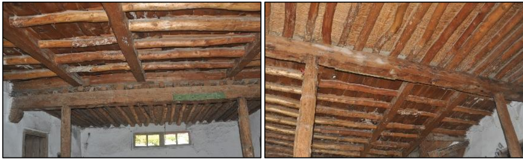
Figure 3.70. Ceiling view of Timber Flooring Type 1 and Type 2 (Cumhuriyet N. b.block-lot:433-2)
