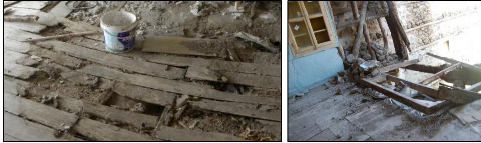
Figure 3.67. View of timber floor boards of flooring of Type 2 used in the room (left, Yenice N. b.block-lot: 521-12; right, Kubbeli N. b.block-lot: 186-36)
