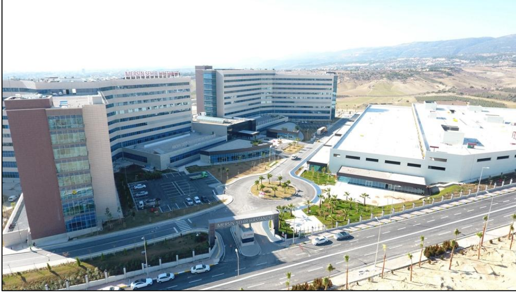
Figure 5.6 Aerial View of Mersin City Hospital (Source: CCN Mersin Sağlık A.Ş.)
