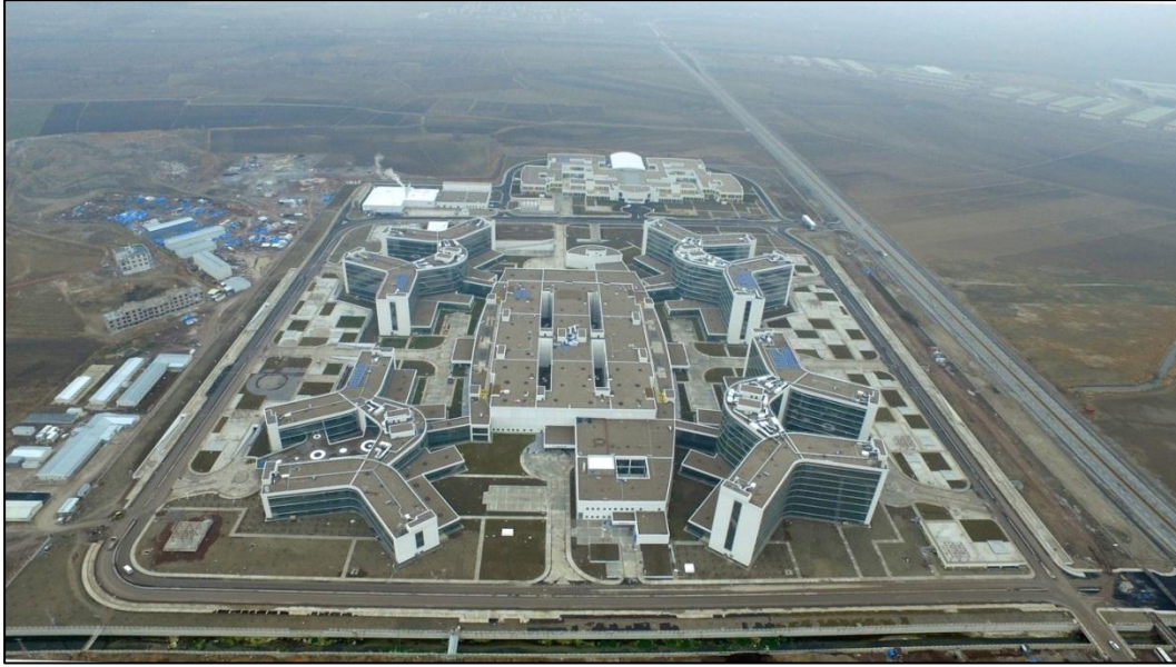
Figure 5.13 Aerial View of Kayseri City Hospital (Source: Kayseri Şehir Hastanesi, 2018)
