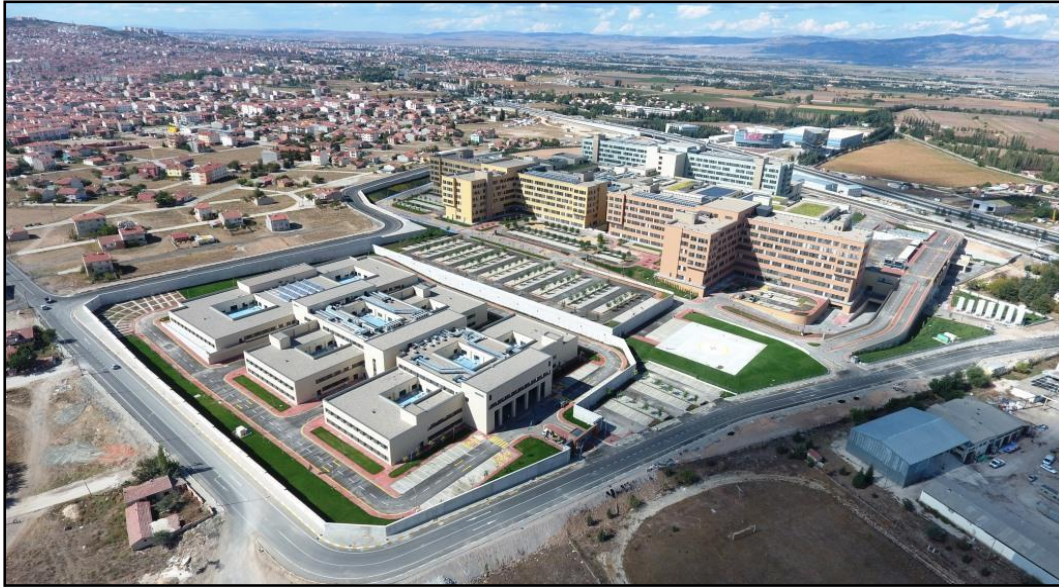
Figure 5.19 Aerial View of Eskişehir City Hospital (Source: Eskişehir Şehir Hastanesi)
