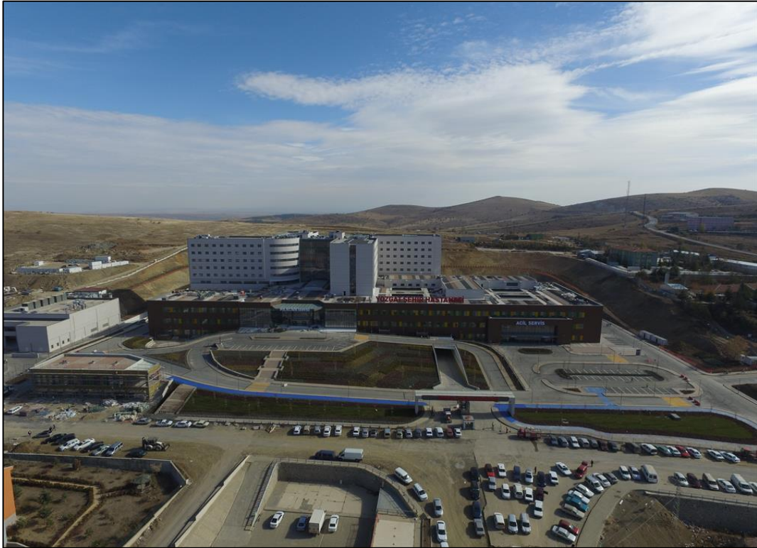
Figure 5.8 Aerial View of Yozgat City Hospital (Source: Yozgat Şehir Hastanesi, 2018)
