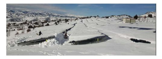
Figure 35- Snow Accumulation on PV Panels-2
