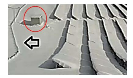
Figure 34- Snow Accumulation on PV Panels-1
