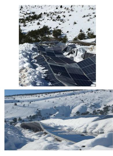
Figure 3- Damaged PV Mounting Structures, Ekol Loss Adjusting (2018)
