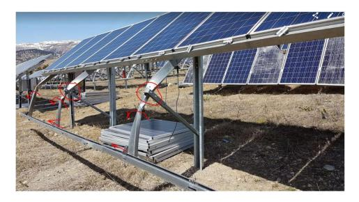
Figure 37- Damaged Main Beam-1
