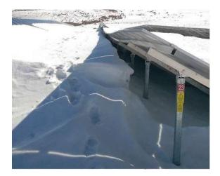
Figure 36- Snow Accumulation on PV Panels-3
