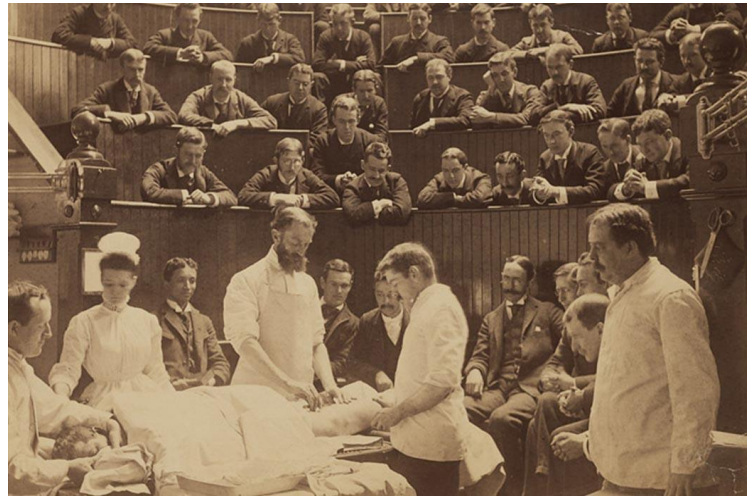
Figure 2.20 Boston City Hospital, Operating Theater, 1890
