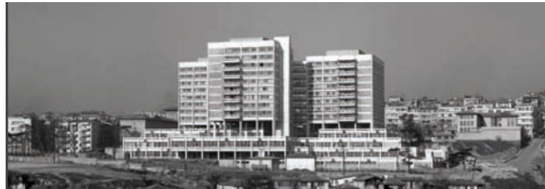
Figure 3.36 Front View, Şişli Children's Hospital
