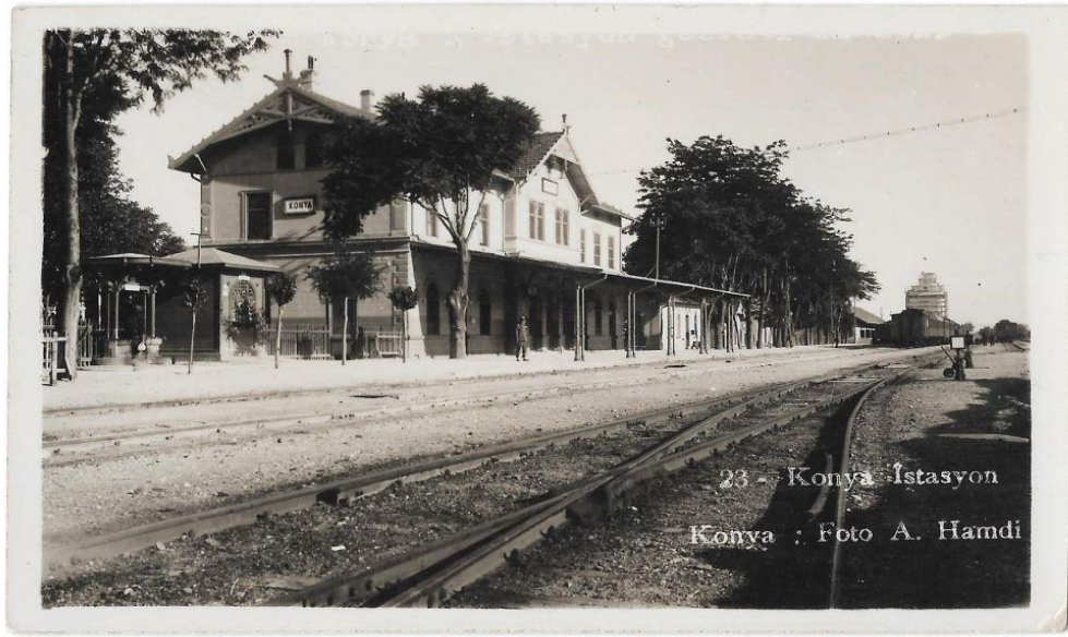
Figure 4.9. Konya old station in past years, platform view. (Showing that canopy has not the same length with the project). (Source: https://www.pingudumuzayede.com/ ) (Accessed 03.12.2019)
