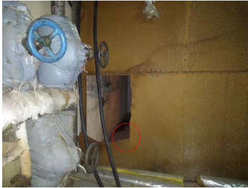
Figure 4.14. The selected area for risk assessment in the Building-E [red circle shows the sampling location]
