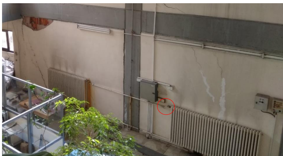
Figure 4.5. The selected area for risk assessment in the Building-B [red circle shows the sampling location]
