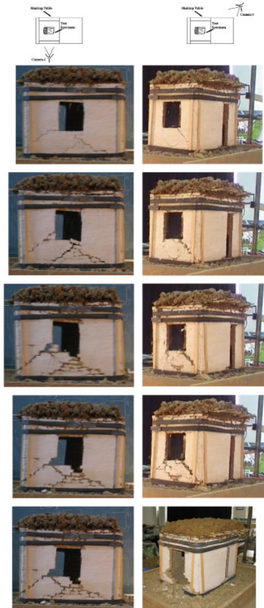
Figure 13. Failure sequence of specimen (HSS2).
