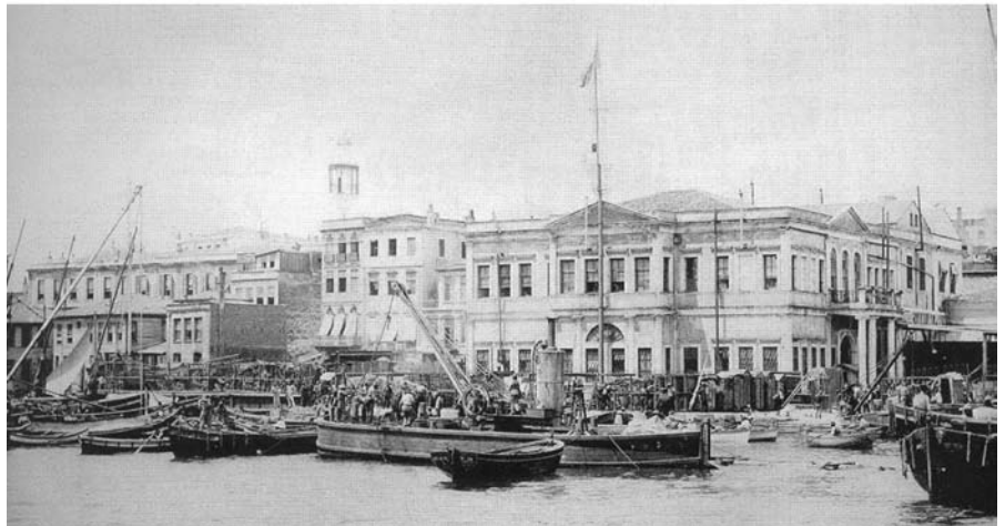
Figure 15.2. The photograph of the customhouse quay after the demolition of the front façade of the Leaded Magazine and the construction of the Public Health Offices, ca.1870-90.
