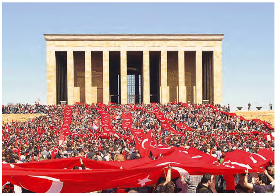
Figure 19. Staircases are exposed to excessive live loads due to ceremonial crowds in national events.
