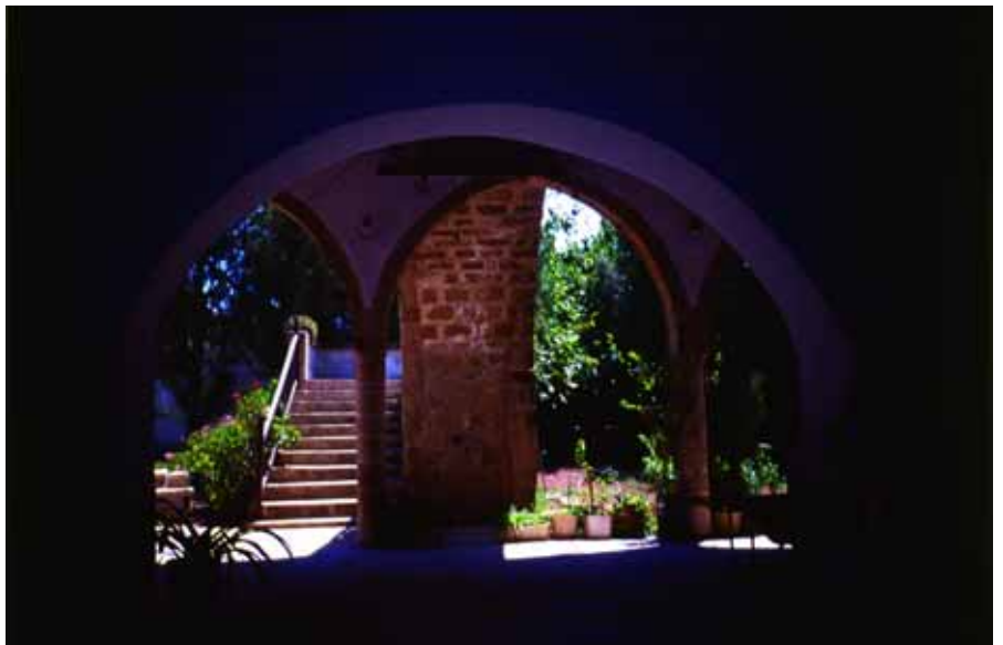
Figure 20. The Wide Arch Entrance Gate towards the School for Girls-I. (B. Özgüven)
