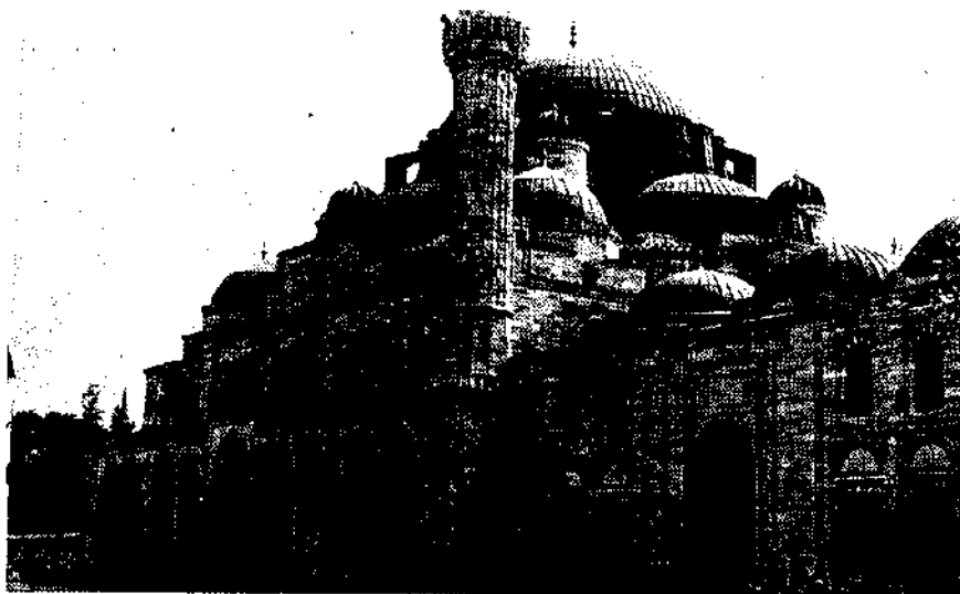
Fig. 2 East Façade of Şehzade Mosque, 1543 - 1548
