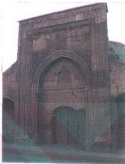
A1.1 Hanikah, Entrance Façade
