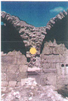
F.4 Courtyard, North Side Vaults ( ● zaz.SM2)
