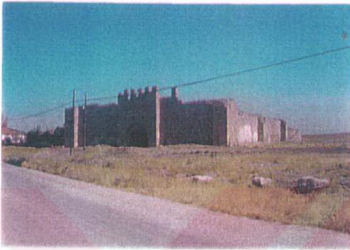
G1. Obruk Han, General View
