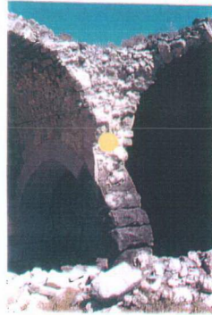
F.5 Courtyard, North Side Vaults ( ● zaz.SM3)
