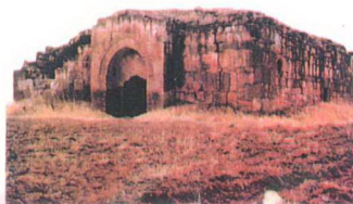
II.2 Mescid Building, General View
