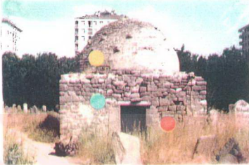
E1.1 Evhadeddin Kirmani Tomb, Entrance Façade (● ev.BM1, ● ev.SM1, ● ev.SM2)
