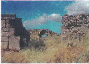
H1. Kuruçeşme Han, Entrance Façade
