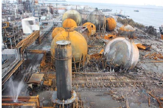
Figure 2.1. Displaced Spherical LPG Storage Tanks (Zama et al., 2012)
