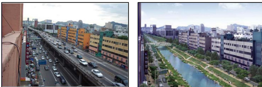
Figure 3.9. Before and After Cheonggyecheon River [Source: Landscape Architecture Foundation (2010)]
