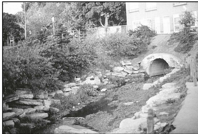
Figure 3.4. In the Strawberry Creek construction, the culverts were reused as steps to improve the stream bank [Source: Gary Mason of Wolfe Mason Associates (1984)]
