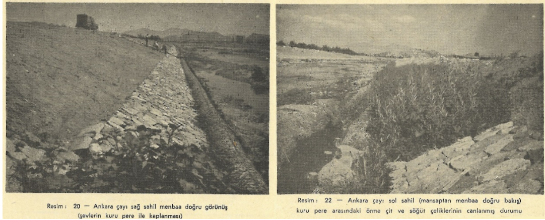
Figure 4.17. Ankara Stream while strengthening with stone filling and plantation
