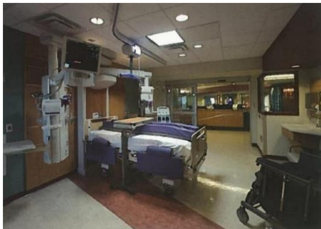
Figure 2.49. The Lancaster general hospital, Wall- mounted pendant life support system, PA, USA (Hamilton & Shepley, 2010, p. 114)
