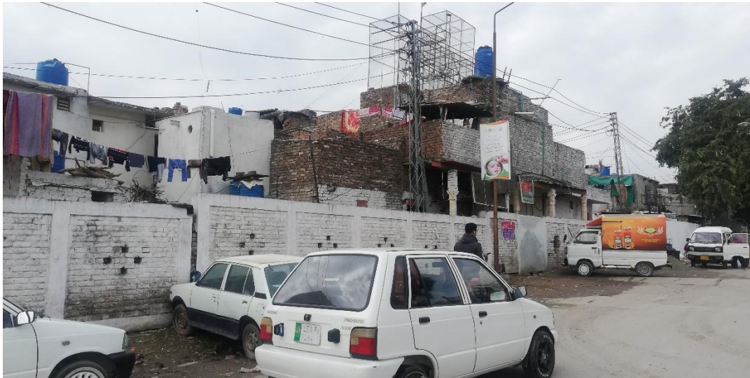
Figure 5.10 Boundary wall of France Colony. Source: Author
