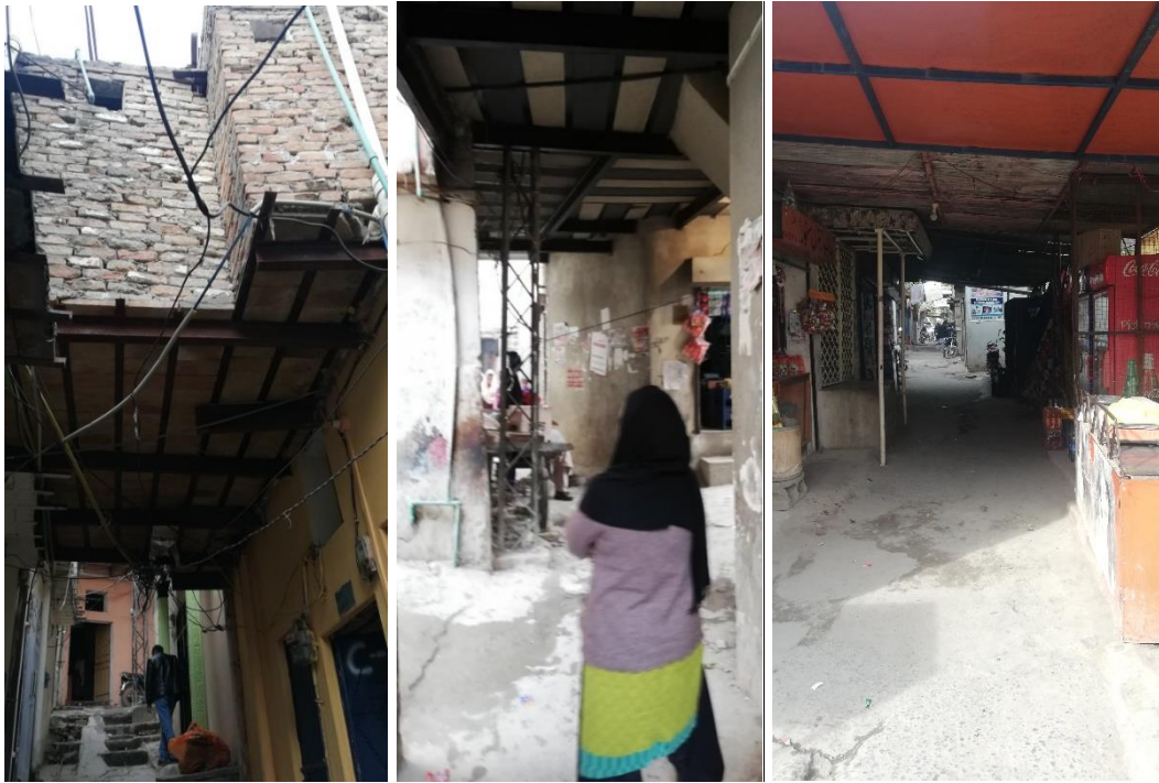
Figure 5.13: Extrusions and levels added to extend the living areas, often hovering over street spaces
