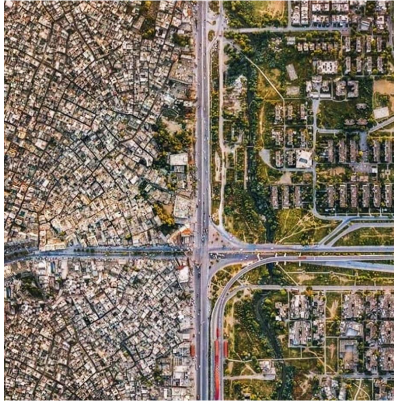
Figure 1.1 Aerial view of the adjacent cities of Rawalpindi and Islamabad with a stark contrast in their urban fabric.
