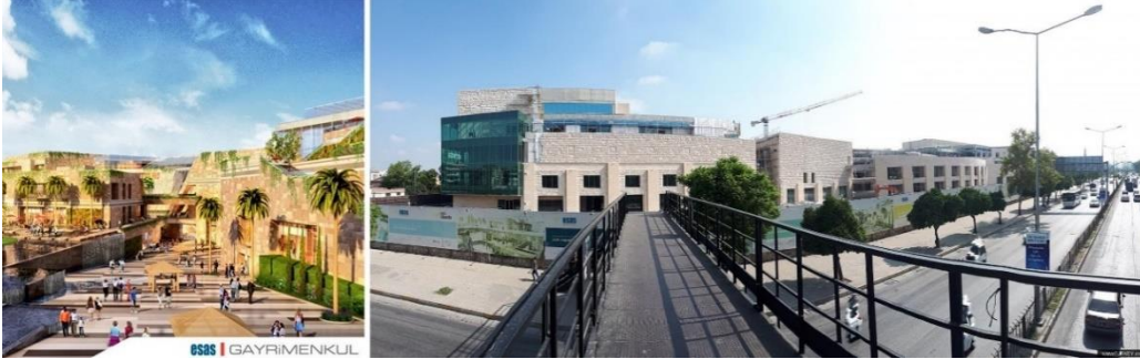
Figure 4.64. project image of the Esas 01 Burada Mall built on the site of old Tekel Factory on the left (Retrieved from http://www.esasgayrimenkul.com.tr/ ) and its construction (Source: author's personal archive)
