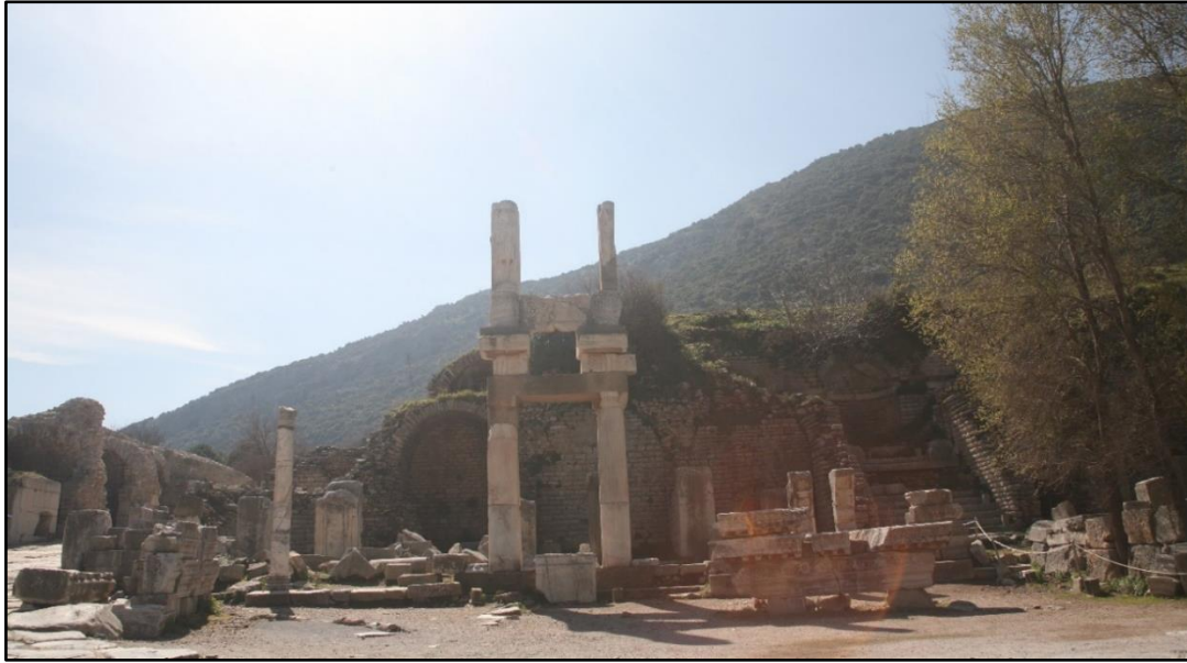
Figure 98 – View of the north façade of the substructures of the Temple of the Sebastoi from the plaza (author’s photograph)
