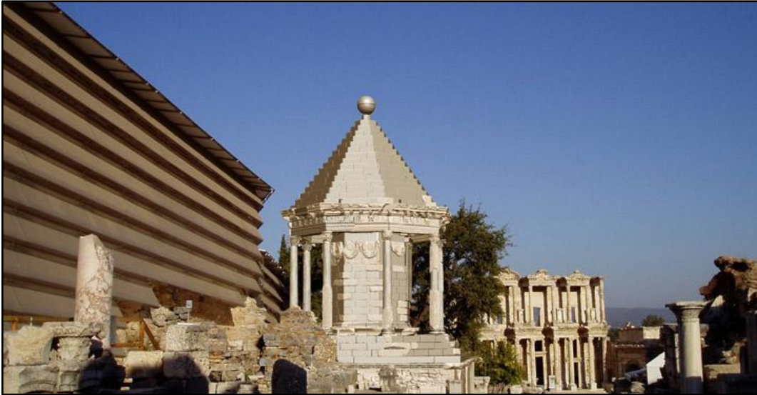
Figure 62 – Reconstructed model of the Octagon placed on its original urban context by ÖAW-ÖAI/B. Thuswaldner
