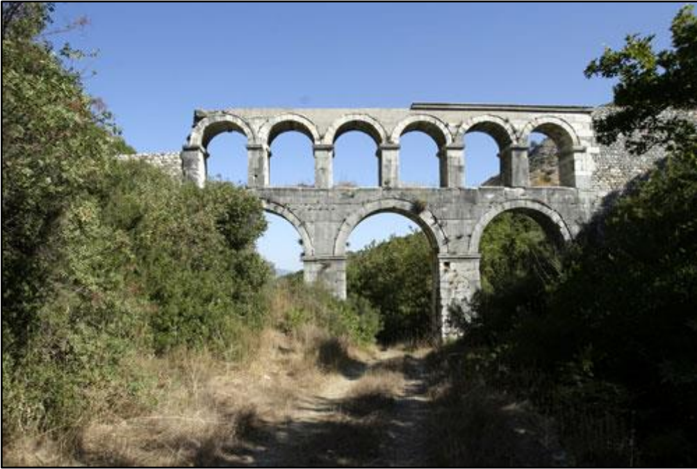
Figure 91 – The Pollio Aqueducts, part of the water conduit called the Aqua Throessitica
