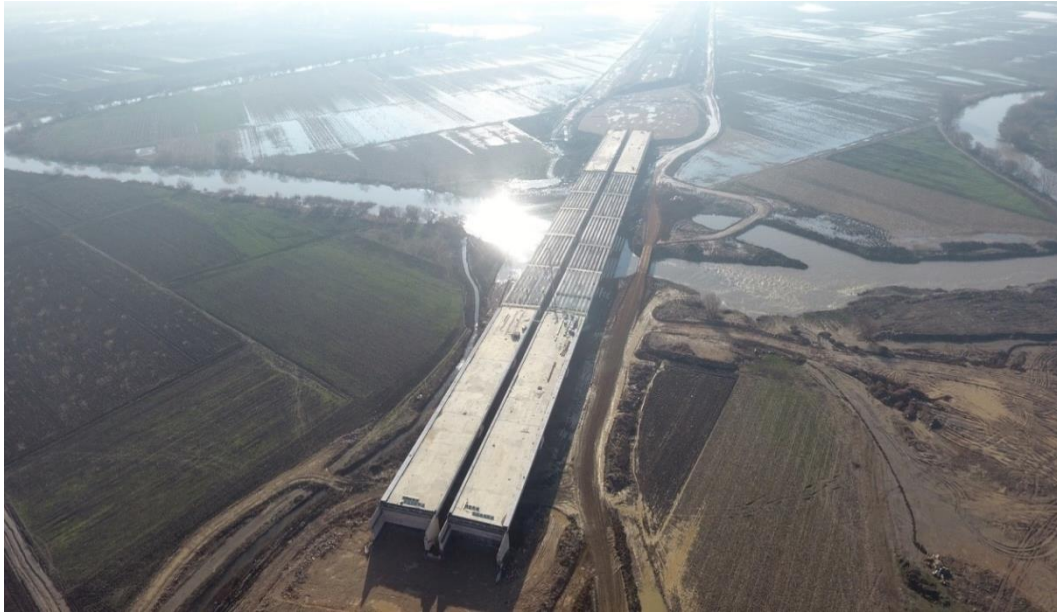
Figure 3.5. Flood plain view of Karacabey Plain
