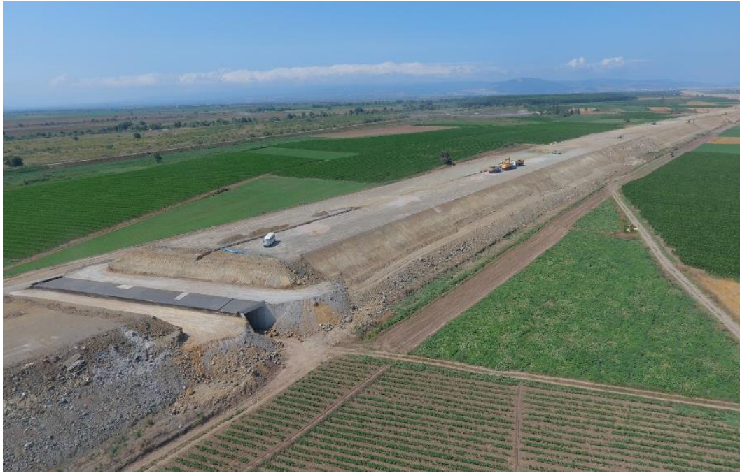
Figure 3.2. Embankment construction on the Karacabey Plain
