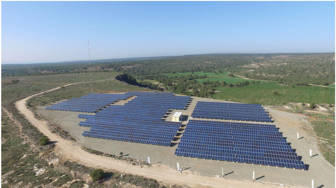
Figure 21. Aerial view of METU NCC solar power plant.
