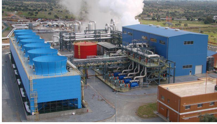
Figure 11: Photo of Germencik Geothermal Power Plant in Turkey (double flash technology with installed capacity of 47.4 MW e ) [36].
