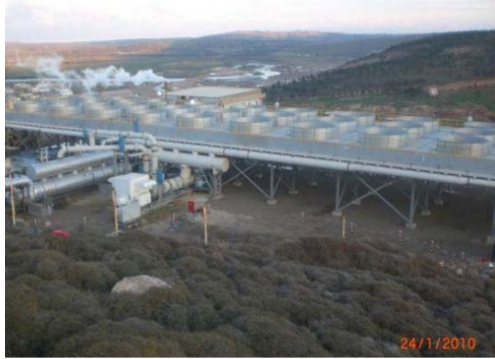
Figure 13: Photo of Tuzla Geothermal Power Plant in Turkey (with installed capacity of 7.5 MW e -Binary cycle) [38].
