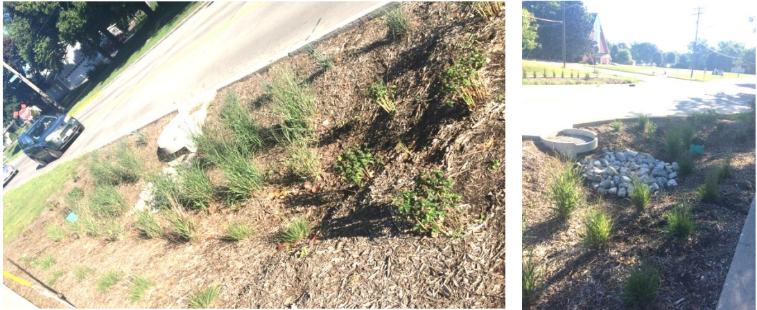
Figure 4. Bioretention in the city of Ames, IOWA, USA.
