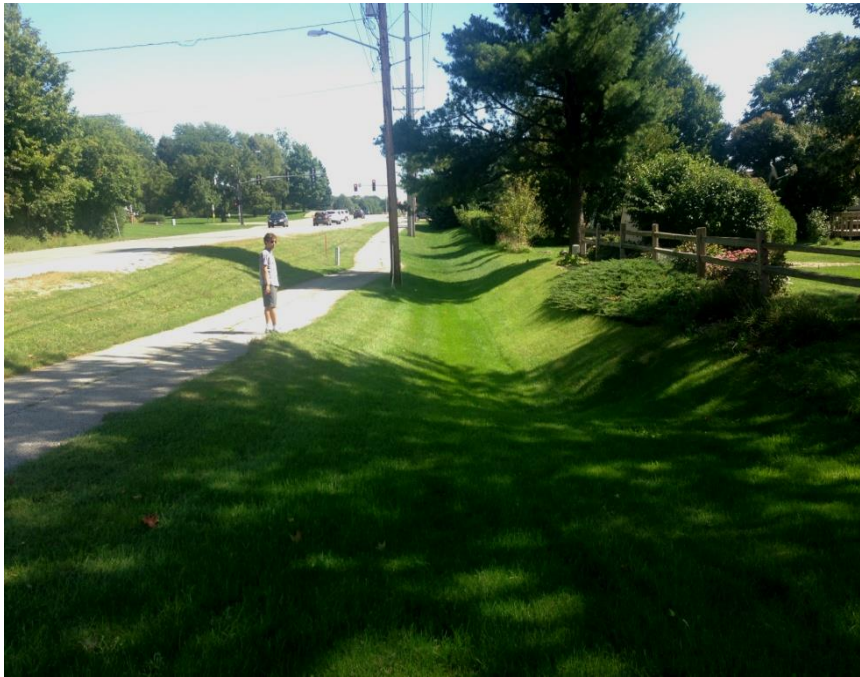
Figure 7. A grass swale in the city of Ames, IOWA, USA.
