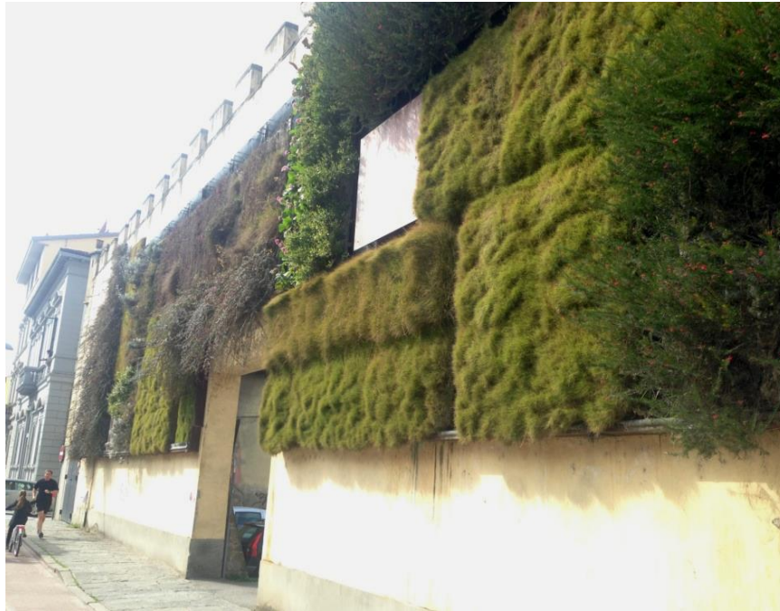
Figure 6. A sample of vegetated wall in Florence, Italy.
