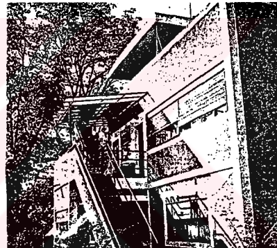
Figure 3.25 The open staircase on the front facade of this detached house was one of Le Corbusier's most attractive ideas. The landing of the staircase was used as verandah and the area beneath the stilts were enclosed, by the tenants.
