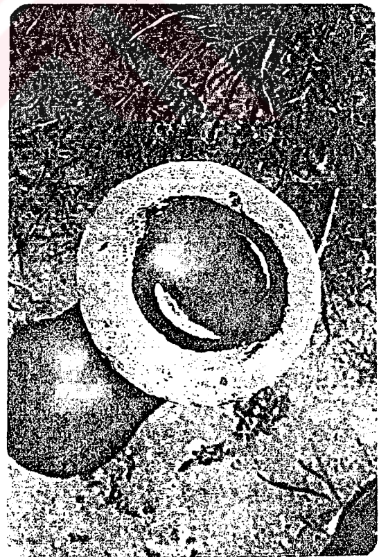
Figure 17f. Original Drainage Pipe of the "Mescid"
