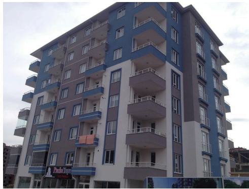
Figure 7. Residential building (C) ( https://earth.google.com , 2020).
