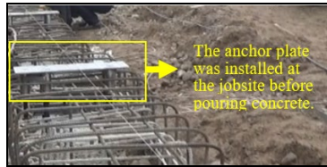
Figure 5a: Anchor plate in the jobsite.
