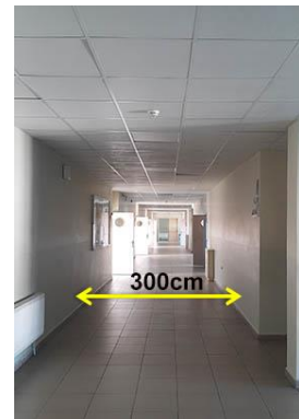
Figure 10: Corridors of classrooms.
