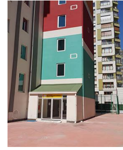
Figure 14: School escape gate.
