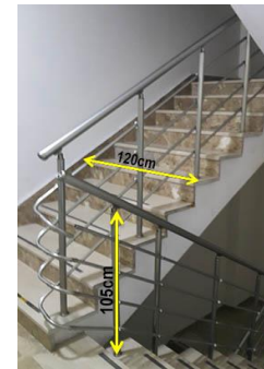
Figure 18: The main stairs.
