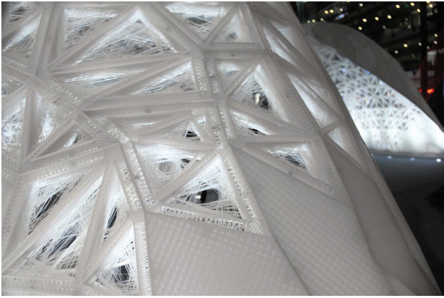
Görsel 9: Beijing's Laboratory for Creative Design'dan Yu Lei ve Xu Feng, Vulcan Pavillion, 1023 farklı modül ( https://www.designboom.com/architecture/vulcan-beijing-design-week-bjdw-largest-3d-printed-architectural-pavilion-parkview-green-10-07-2015 ). (ET:02.06.2020)
