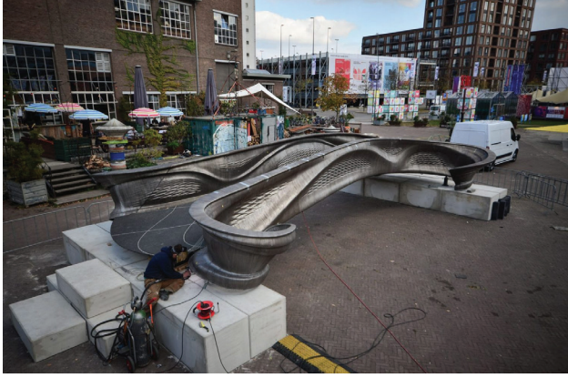
Görsel 10: MX3D ve Arup, Paslanmaz Çelik Köprü ( https://www.dezeen.com/2018/04/17/mx3d-3d-printed-bridge-joris-laarman-arup-amsterdam-netherlands/ ). (ET:02.06.2020)
