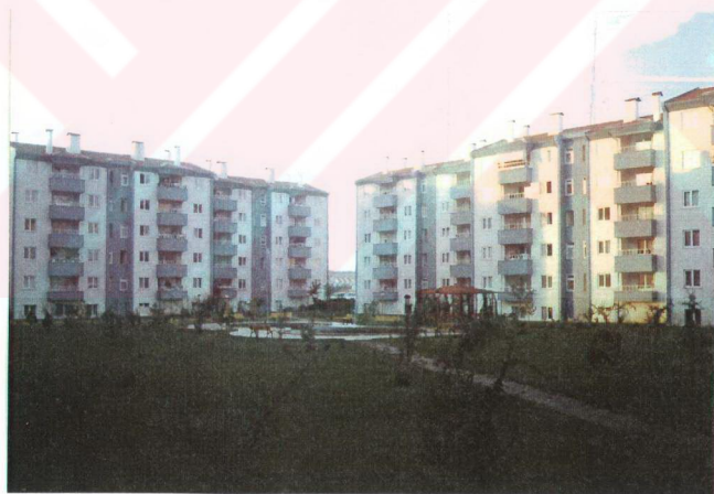
Figure 5.23. The Courtyard: Located in the center of the apartment blocks
