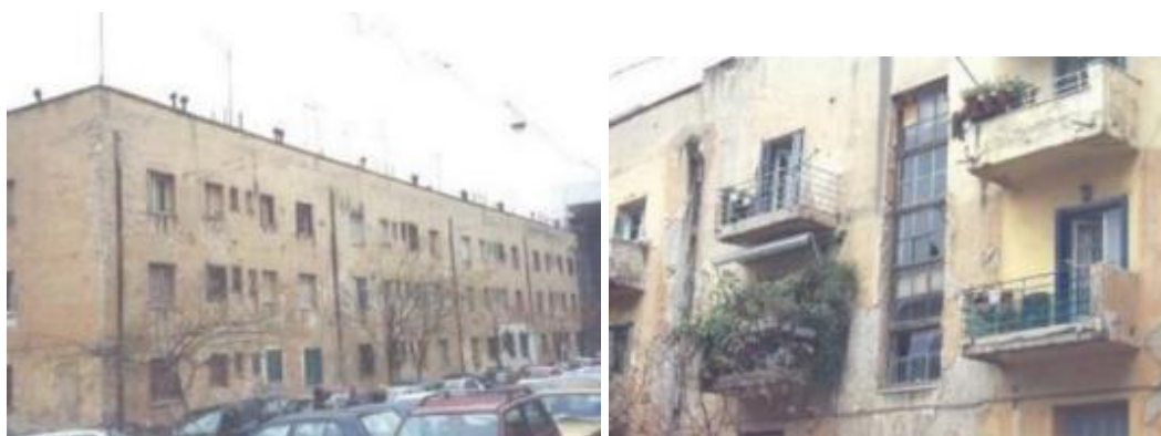
Figure 3.5 Alexandras Prosfygika refugee housing complex in Athenian neighborhood. (Source: https://inura08.files.wordpress.com/2008/09/alexandras_en_.pdf )
