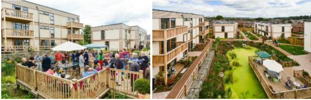
Figure 3.7 Lilac Co-Housing Project – Leeds, UK (Source: https://www.modcell.com/news/lilac-official-opening/ )
