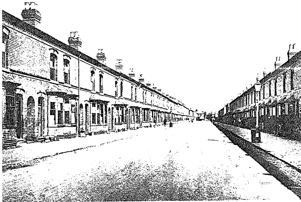
Figure 3.32 Continuous buildings along street A History of Architecture, 681.
