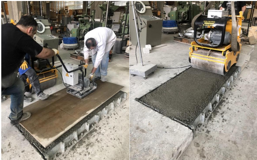
Figure 3-8 Two-steps compaction procedure. Left: initial step; plate compactor, Right: final step; hand roller compactor.
