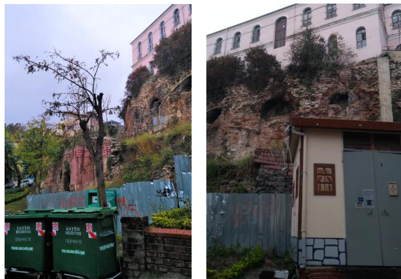
Figure 93. Sultanahmet, current functions surrounding the immediate vicinity of the area, (e.g. the retaining wall, transformer, fencing, rubbish bins, and playground)
