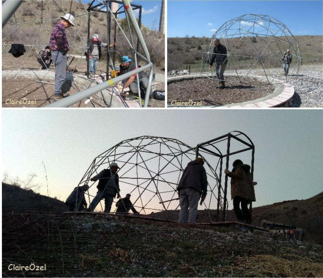
Figure 4.7 The construction process of geodesic dome (Güneşköy, 2021).
