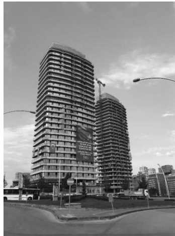
Figure 4.7. Construction site of Togo buildings a conflict site in Ankara (Author, 2019)
