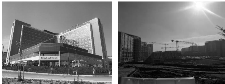
Figure 4.65. Bilkent city hospital and Etlik city hospital construction site in Ankara (Author, 2019: 2018)
