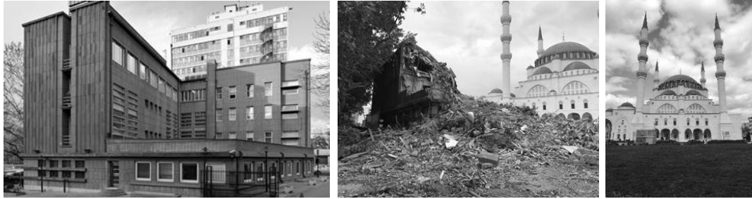
Figure 4.60. Building of İller bank that have cultural, historical, architectural assets; the destruction of building; area after the demolition (Source: Arkiv, 2017; İplikçi E., 2017; Author, 2019)
