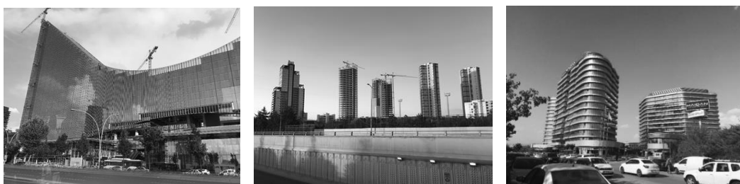
Figure 4.68. Some illustrative figures for office and shopping mall complexes, mixed-used blocks in Ankara (Author, 2019; 2018; 2019)
