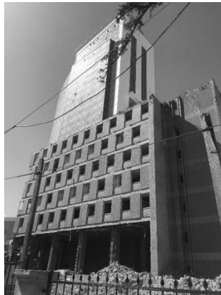
Figure 4.61. Ruins of old and new constructed building of TUIK (Author, 2019)
