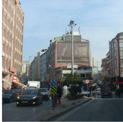
Figure 12: Redeveloped Talatpaşa (Source: www.wikipedia.org )
