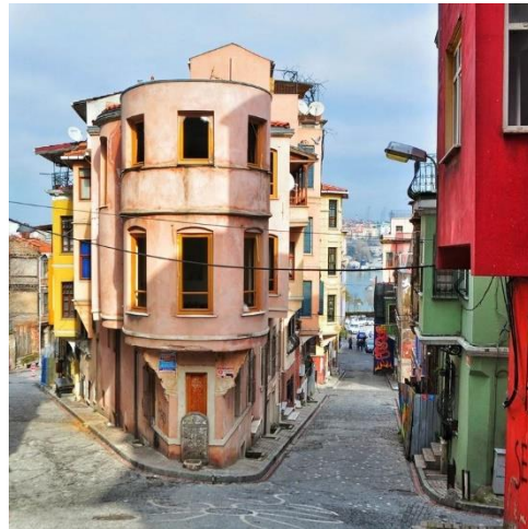
Figure 6: Redeveloped Cibali (Source: www.ekdergi.com )
